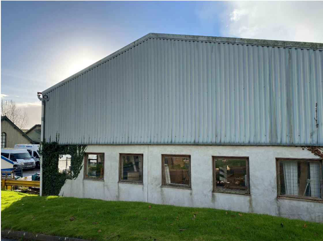
Figure 2: View of East elevation of old engineering workshop
