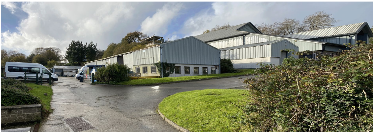
Figure 1: View of South-East elevations of old engineering workshop.
