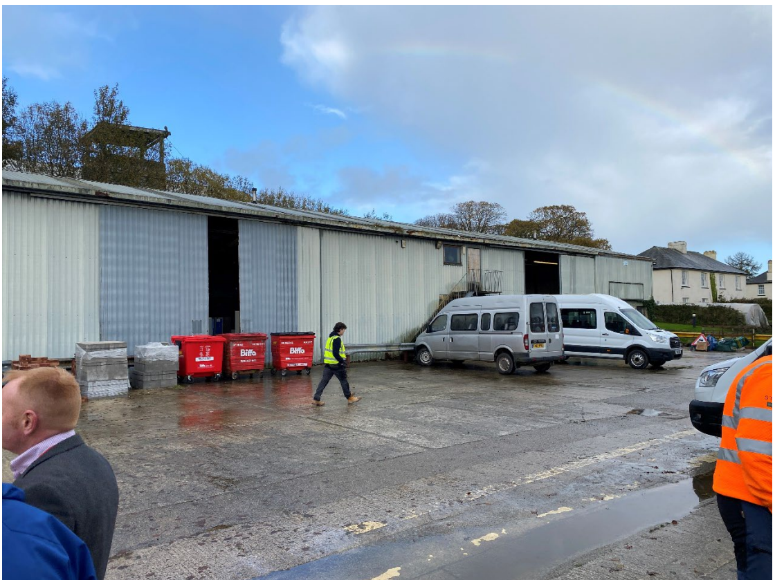
Figure 3: View of South elevation of old engineering workshop
