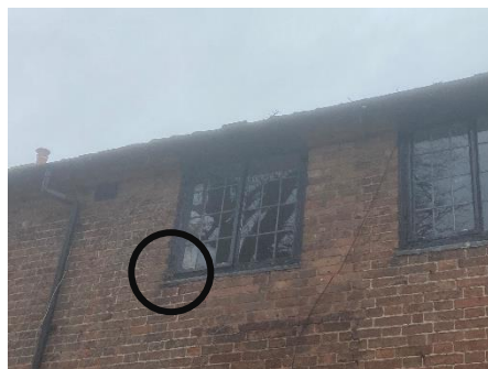
Figure 6- Some windows feature pin hinges suggesting shutters were present prior to the window being installed
