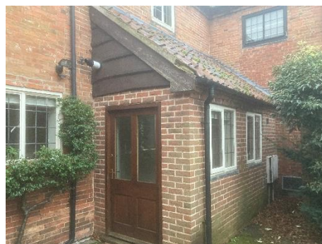
Figure 5- Single storey extension granted permission in 1995
