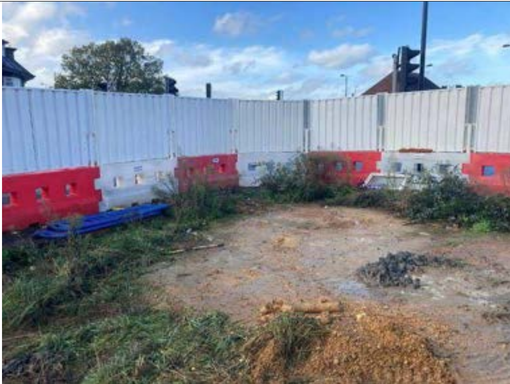
Photograph 2- Hardstanding concrete, in the north of the site. Facing northwest
