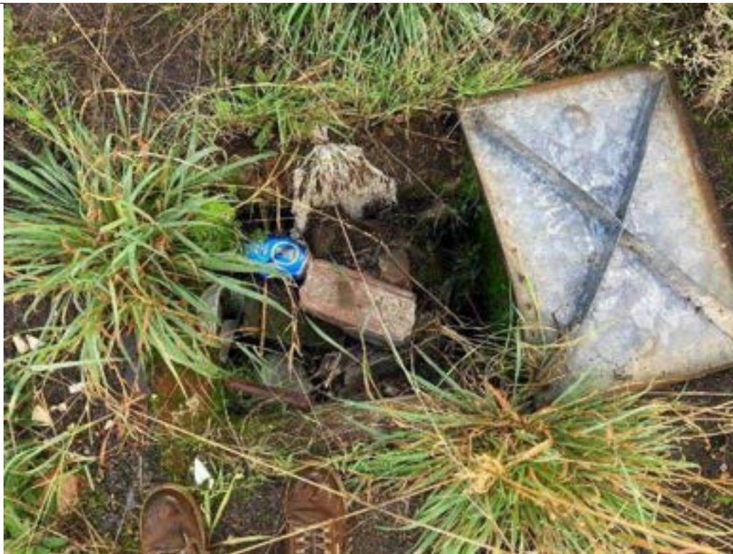
Photograph 4- Exposed manhole cover, presumed drainage.
