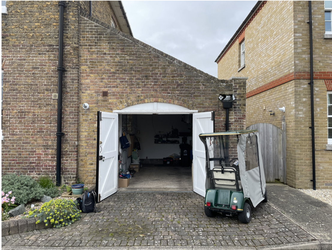
Photograph showing garage doors, to be closed and sealed shut to keep appearance of a garage
