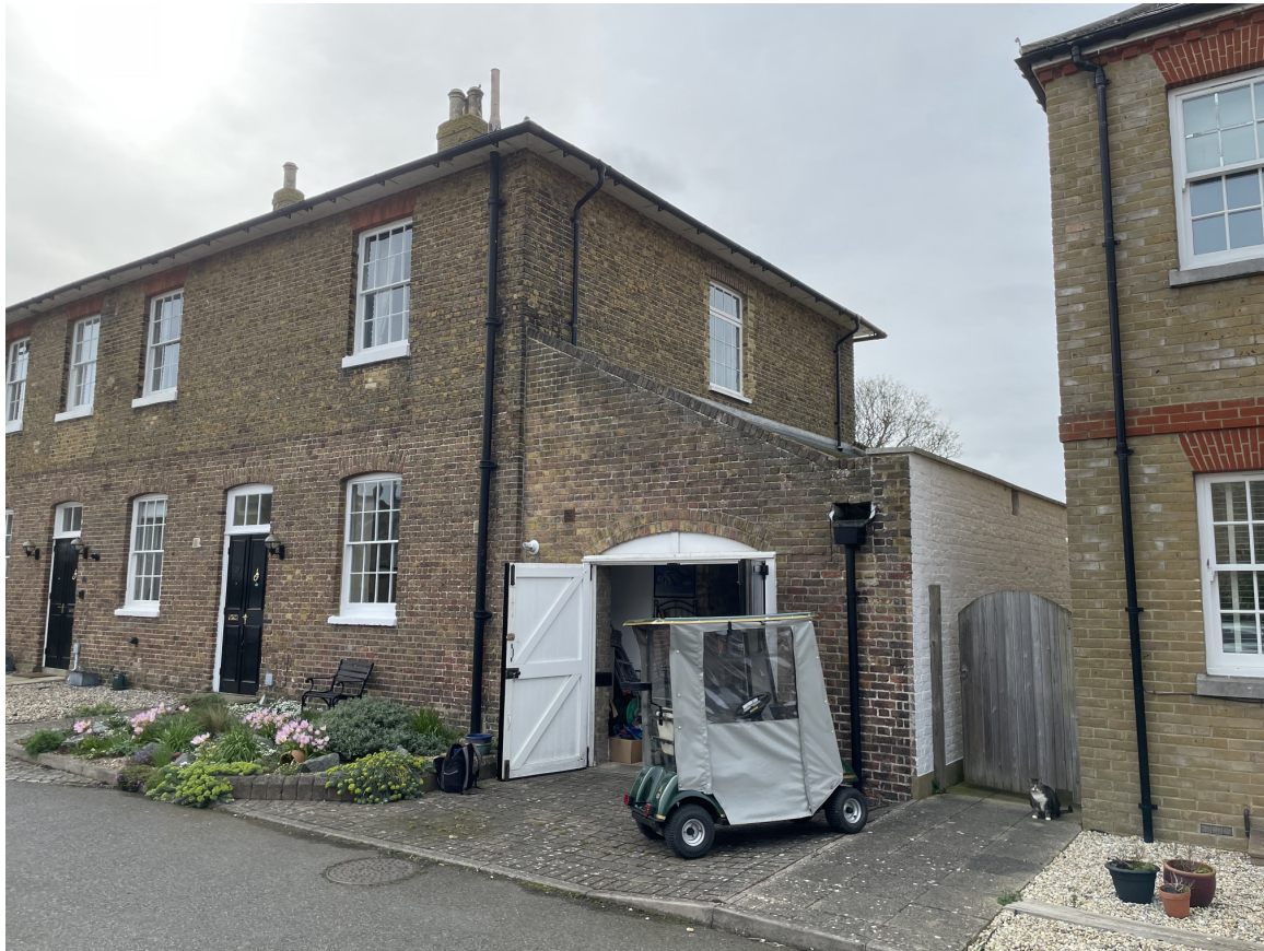
Photograph showing front of garage/dwelling
