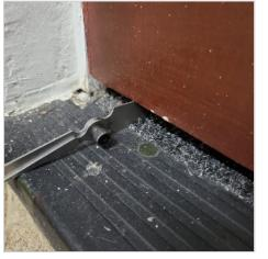
Extensive gaps around door. Extensive gap (16mm) to the topside of the door. Extensive gap (19mm) to the underside of the door. Intumescent seal worn out/painted over. Hinges painted over. Hinges of unknown grade. Hinges leaking oil.
