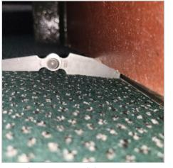
Extensive gaps around door. Extensive gap (9mm) to the topside of the door. Extensive gap (18.5mm) to the underside of the door. Intumescent seal worn out/painted over. Frame damaged beyond repair.
