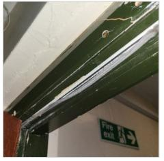
Extensive gaps around door. Extensive gap (14mm) to the underside of the door. Intumescent seal worn out/painted over. Hinges painted over. Hinges of unknown grade. Frame damaged beyond repair.
