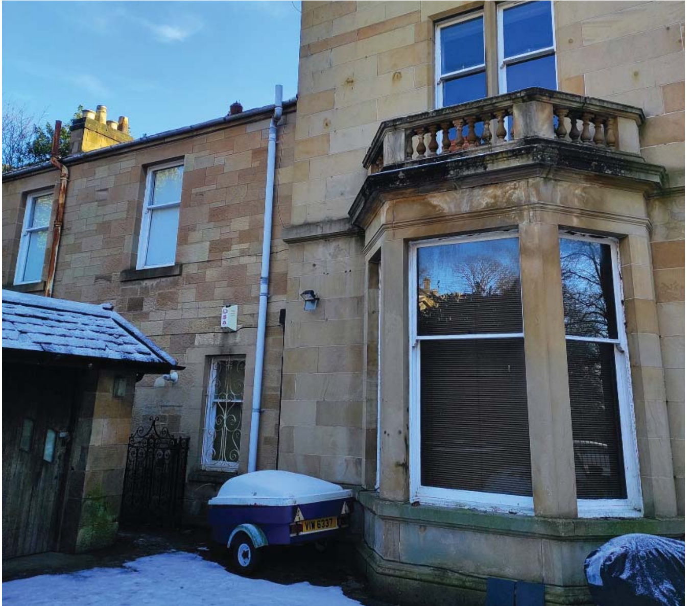
View of the property from driveway
