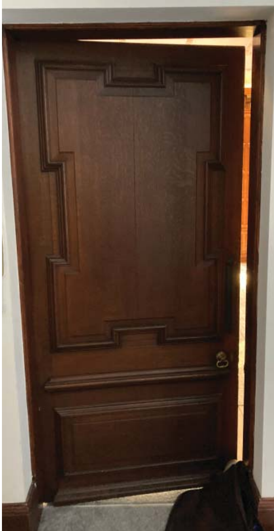
Sitting Room Door (To be nailed shut)
