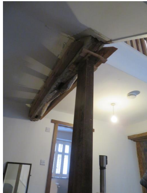
View of beam from below
