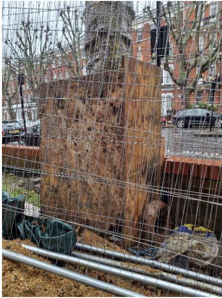
Figure 1 - Plyboard protecting tree trunk
