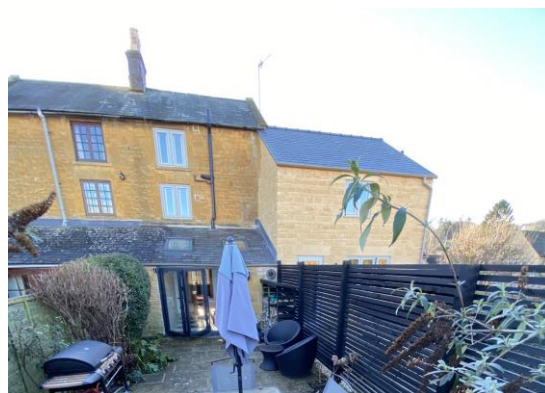
The existing rear elevation which will remain unchanged
