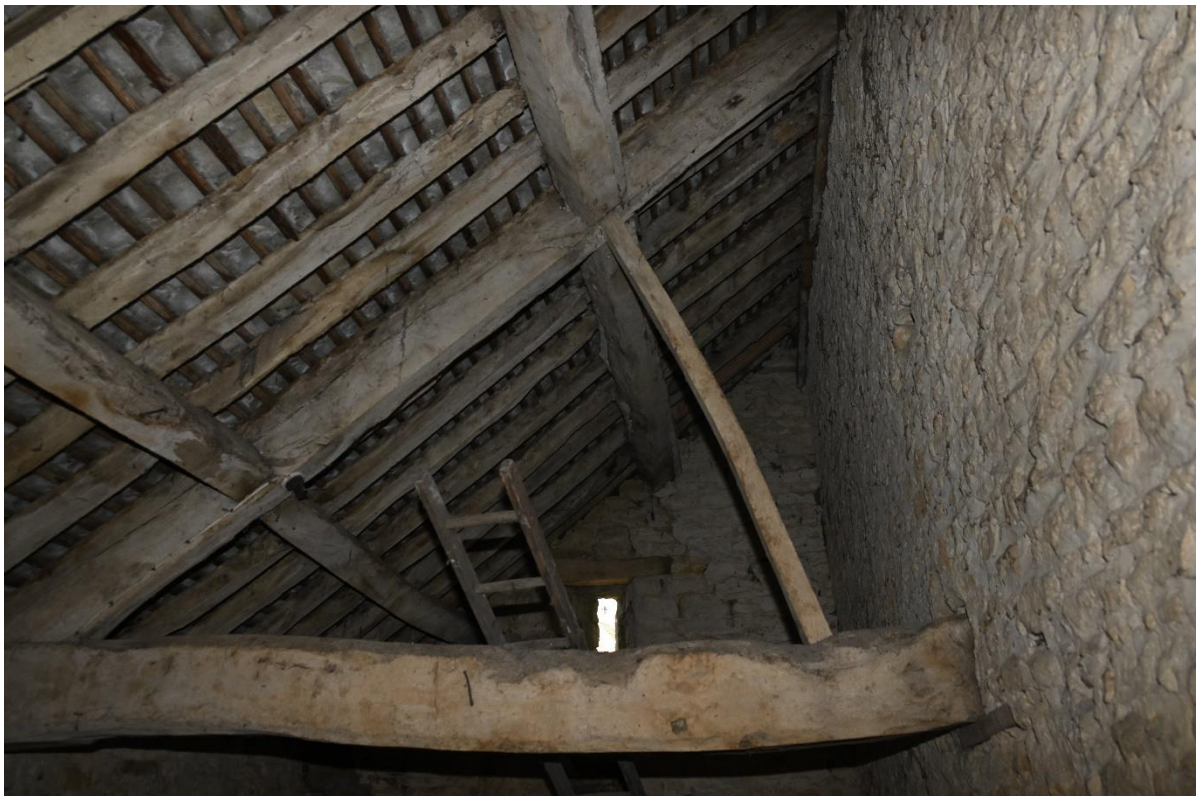
Image 6 Internal structure of lean to building attached to right-hand barn
