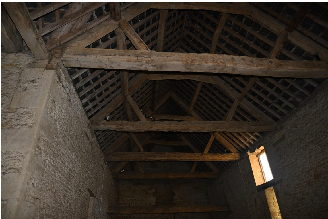
Image 2 Internal structure of left-hand barn
