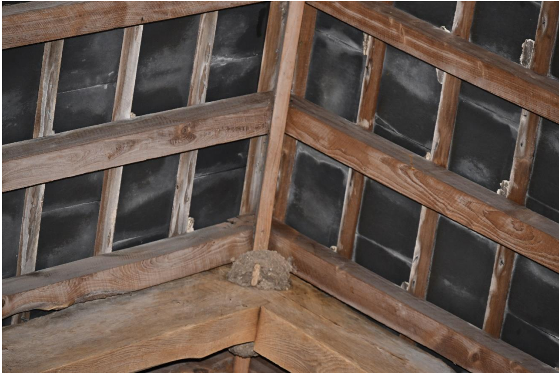
Image 3 Roof structure of left-hand barn
