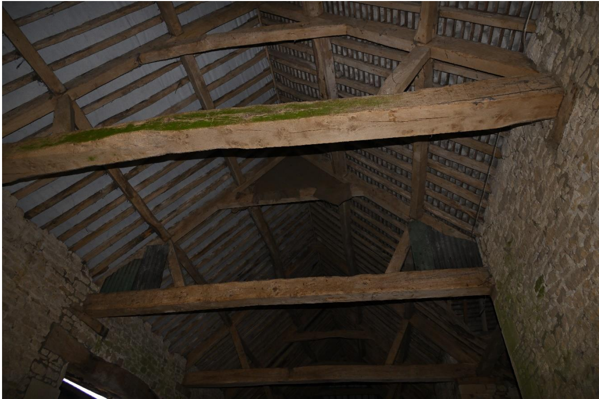
Image 5 Internal structure of right-hand barn – note slightly less ambient light
