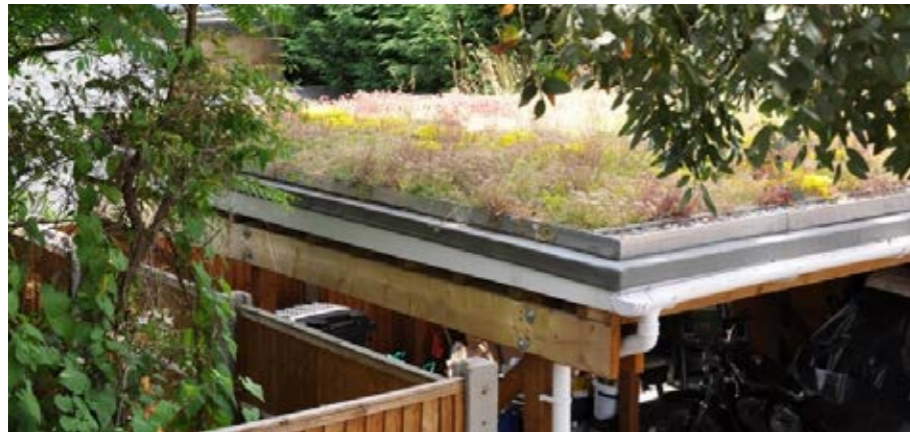
Green sedum flat roof example
