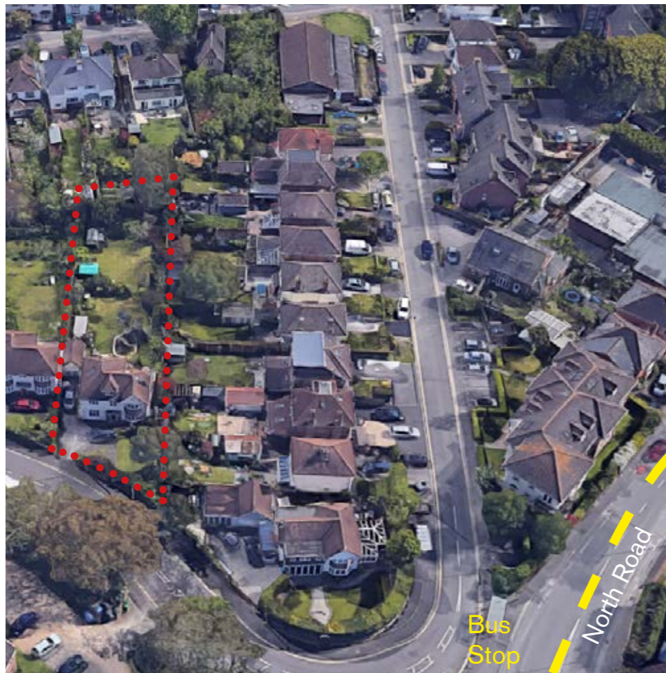
Application site (red dotted line) 3D aerial looking south. Credit: Google Maps
