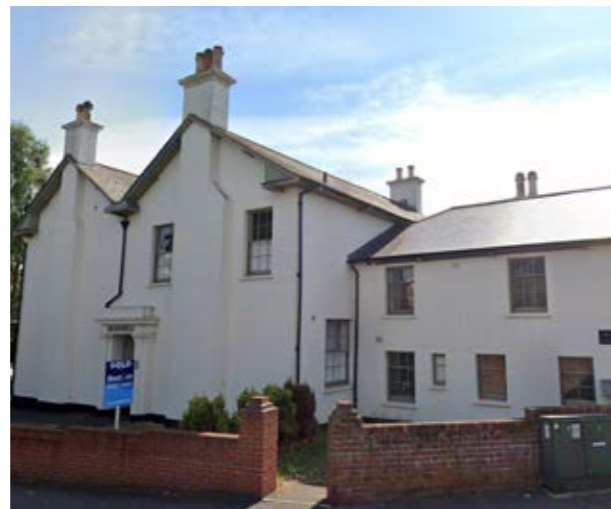
Flats on Danecourt Road / St. Peter's Road Source: Google maps - Change of use granted from commercial to residential. Density of site increased
