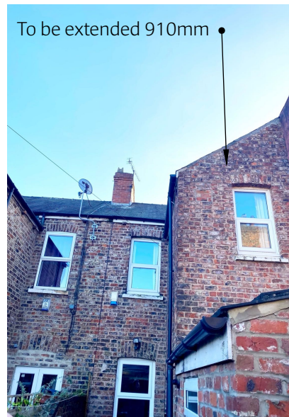
Rear of nos. 15 + 17 Shipton Street
