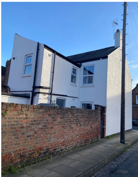
Rear of no. 19 Shipton Street
