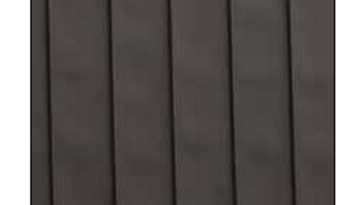
New walls (FF) & roof: Standing seam zinc
