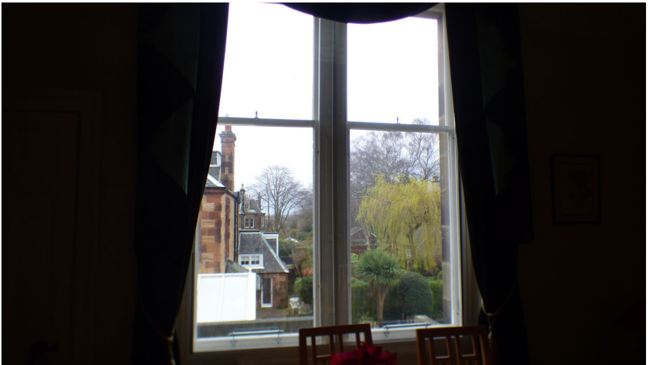
Photograph 3: Showing internal view of Window 1 and 2.
