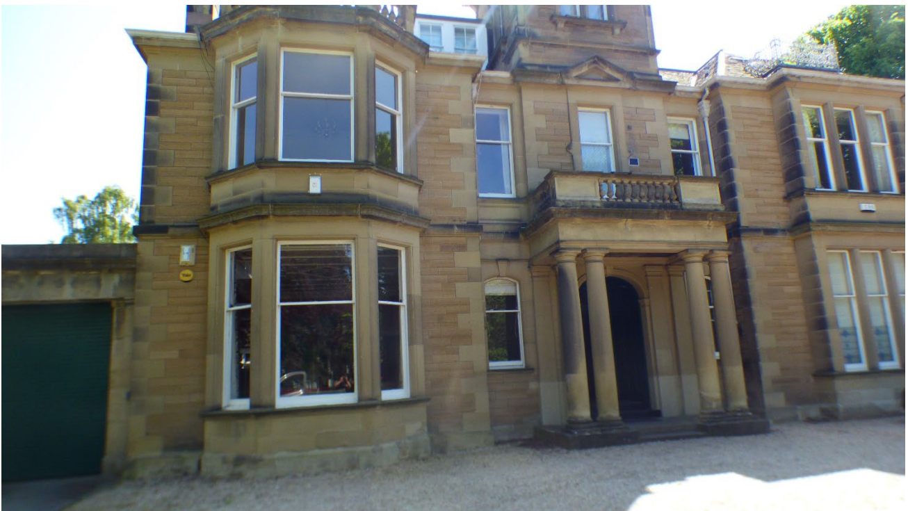
Photograph 1: Showing Front Elevation of 27/3 South Oswald Road, Edinburgh, EH9 2HH.
