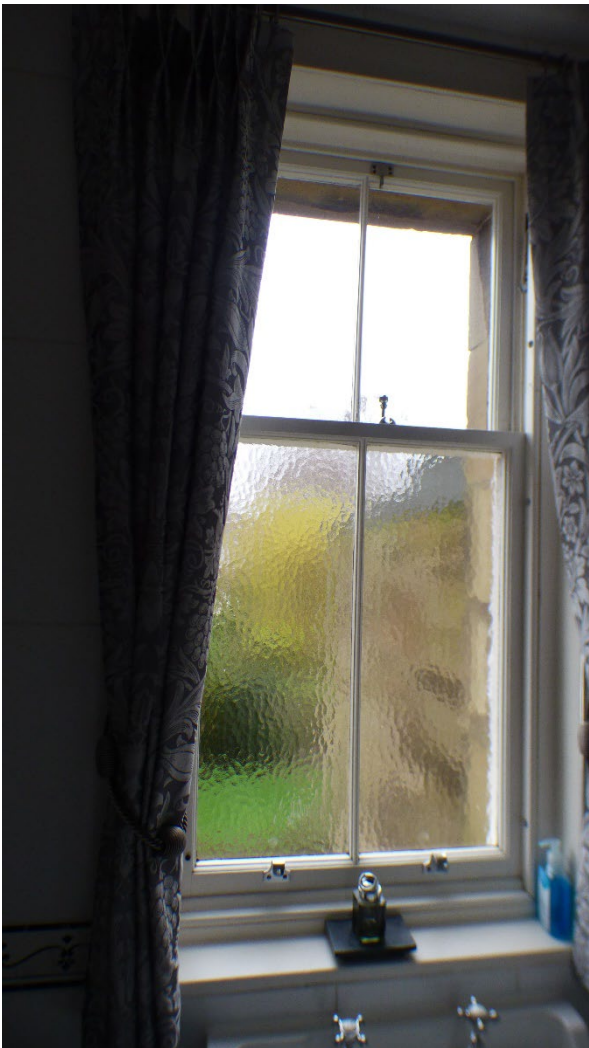
Photograph 19: Showing internal view of Window 4.
