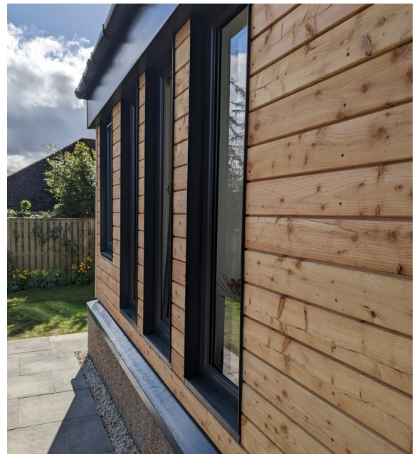
Scottish larch Cladding & high spec Windows
