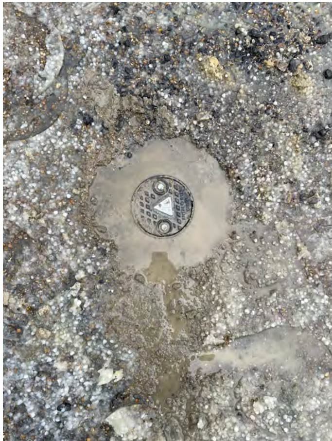
Photo 12—Example reinstatement of borehole
