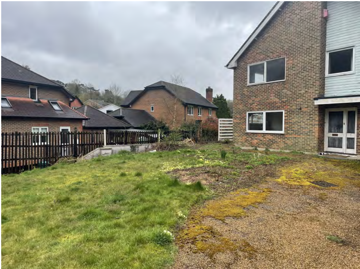
Photo 3—View of the building centrally to the site and retaining wall to the east
