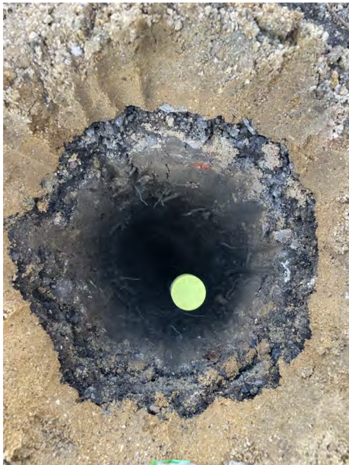
Photo 8—Example view of borehole with pipe install
