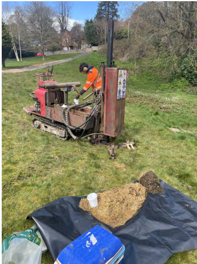
Photo 5—Example of the rig set up at borehole location 5
