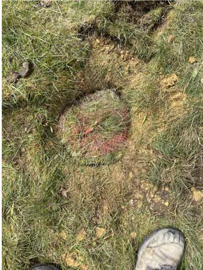
Photo 11—Example backfilled exploratory hole
