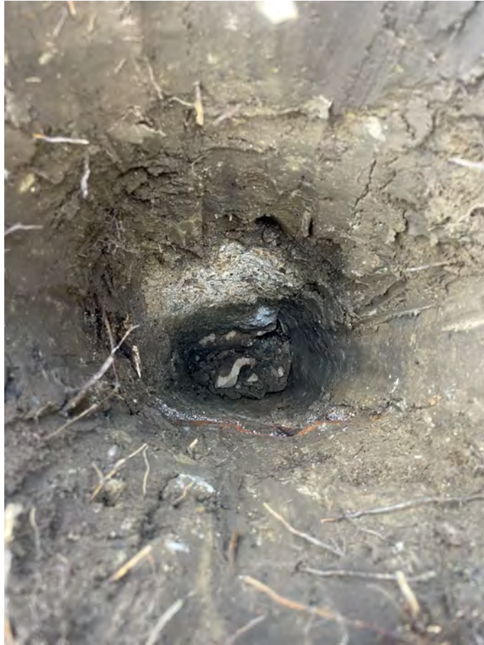
Photo 7—Example view of hand dug safety starter
