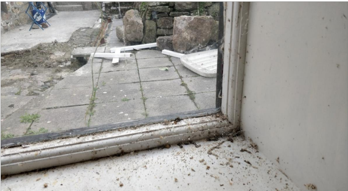
Fig 04 - Former windows – single pane, single-glazed, un-opening, with machined frames.
