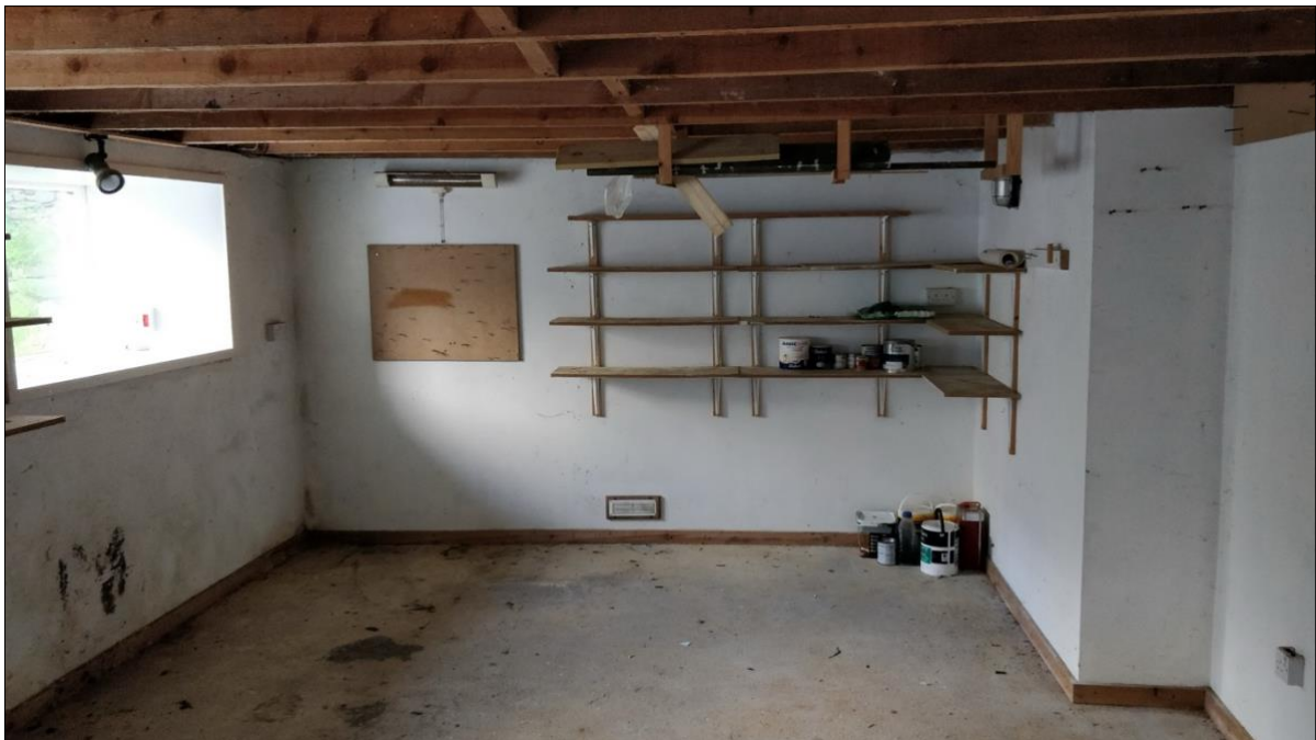
Fig 05 - Internal view showing existing features with modern materials and finishes
