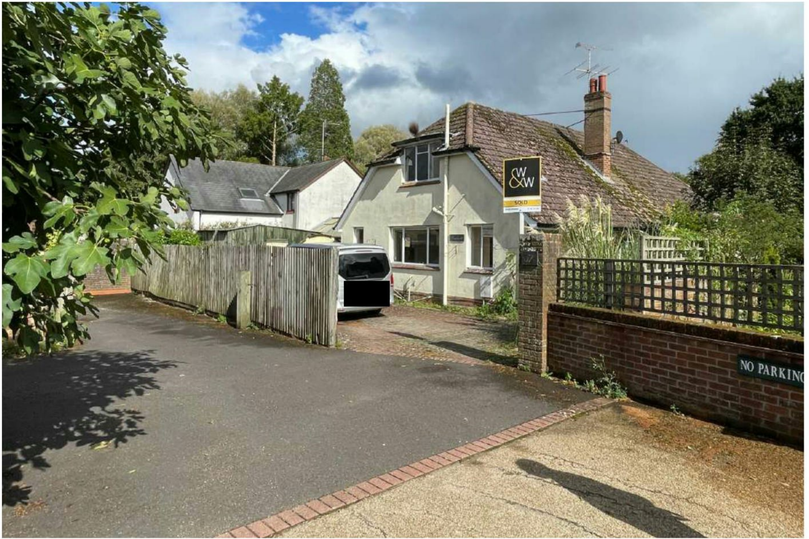
Existing Entrance View
