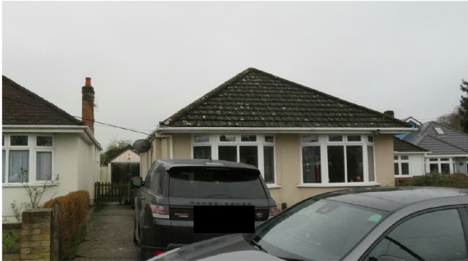
Photo viewing Front / Side of Property from Drive (Camera Facing South)
