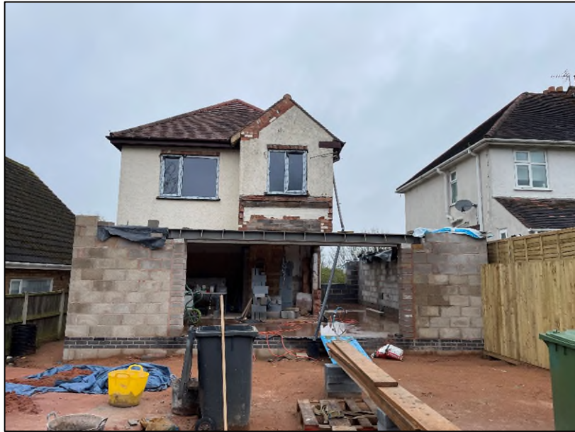
Plate 2: view of the rear of the property. Photograph looking west.
