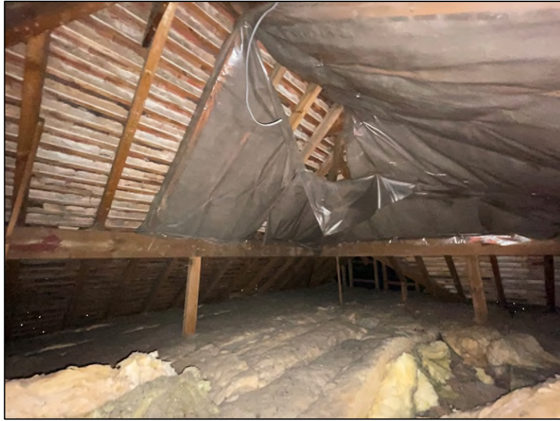
Plate 4: view of the loft. Photograph looking west.
