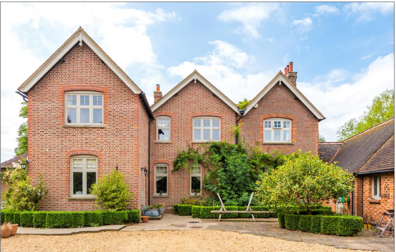
North (rear) elevation of dwelling, facing the highway
