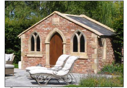
Proposed brick and stone details and slate roof as shown on photo.
