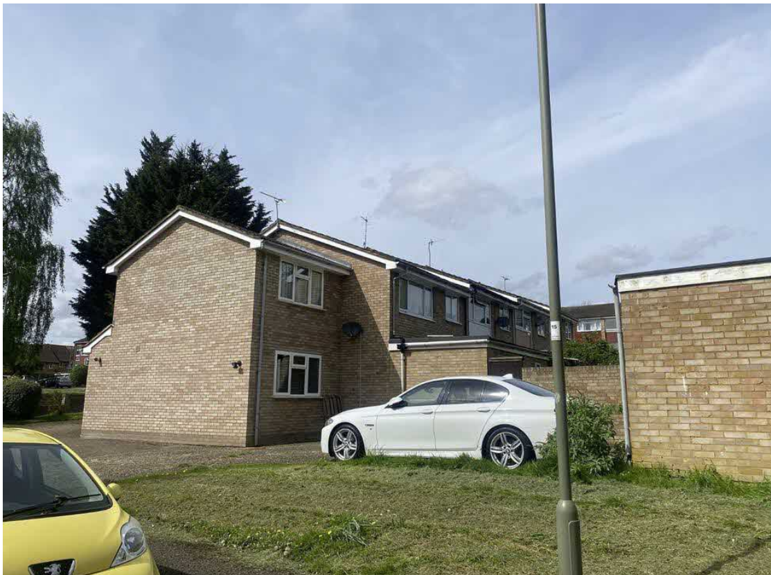
REAR OF 52 - 58 CROMER ROAD
