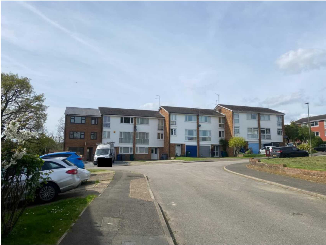
FRONT OF 35A, 35, 37, 39, 41, 43 AND 45 CROMER ROAD
