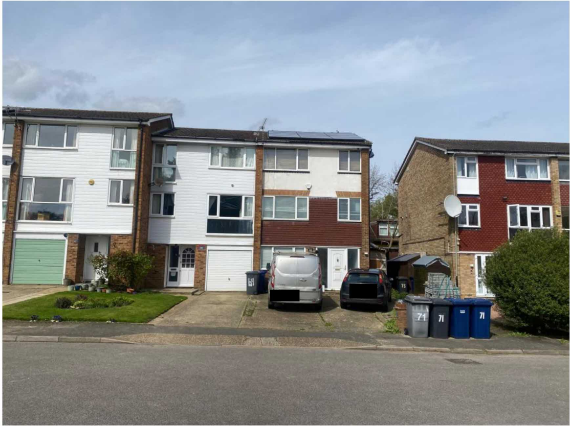
FRONT OF 67 - 73 CROMER ROAD
