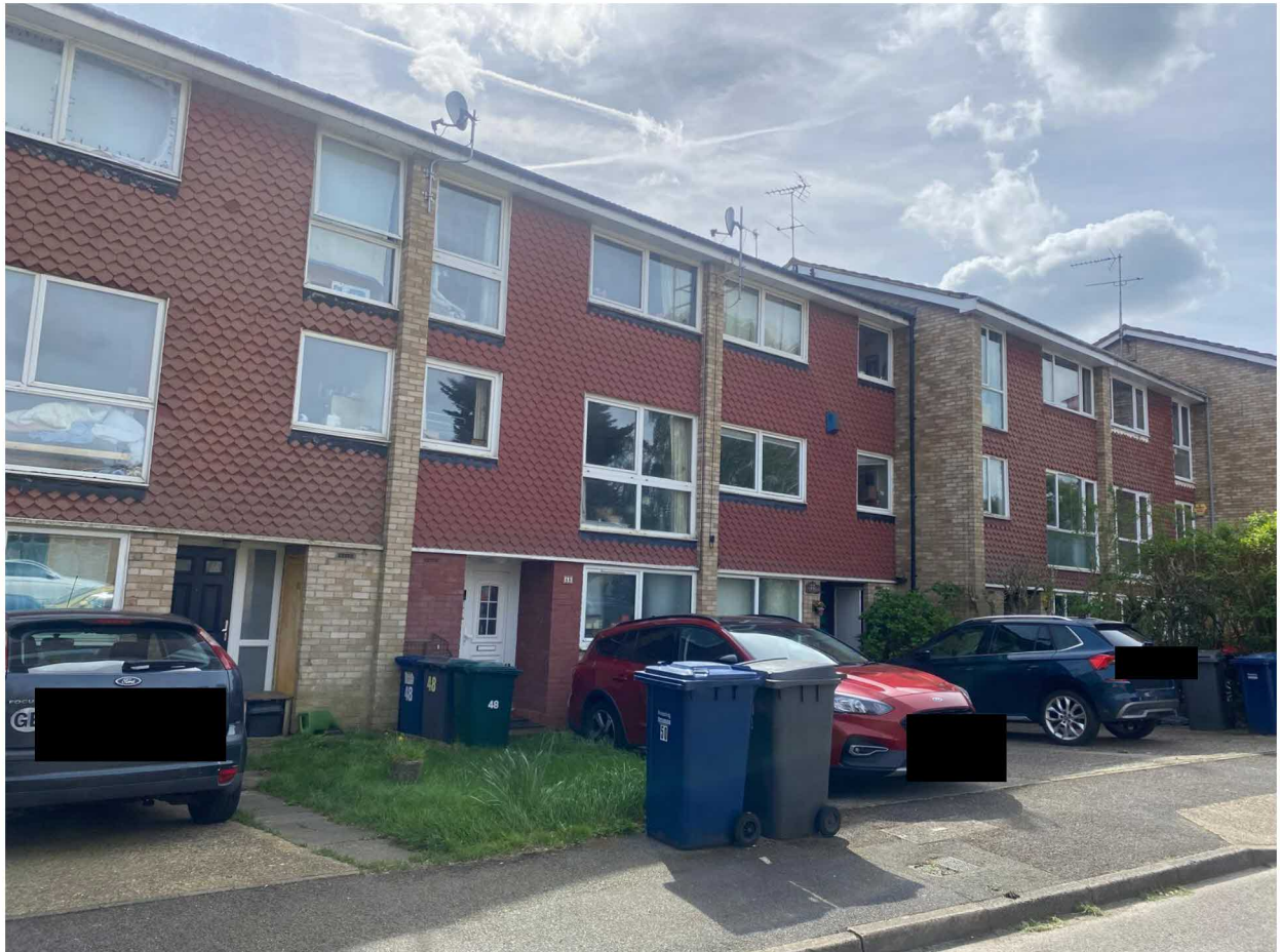
FRONT OF 42 - 50 CROMER ROAD
