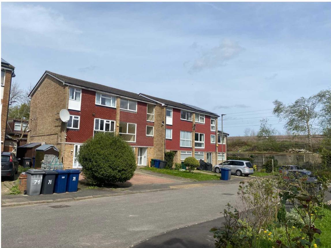
FRONT OF 73 - 79 CROMER ROAD
