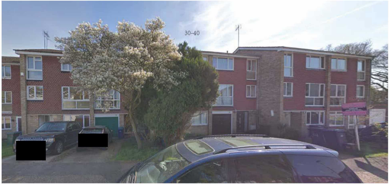
FRONT OF 30 - 40 CROMER ROAD
