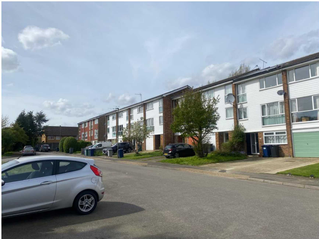
FRONT OF 47 – 67 CROMER ROAD
