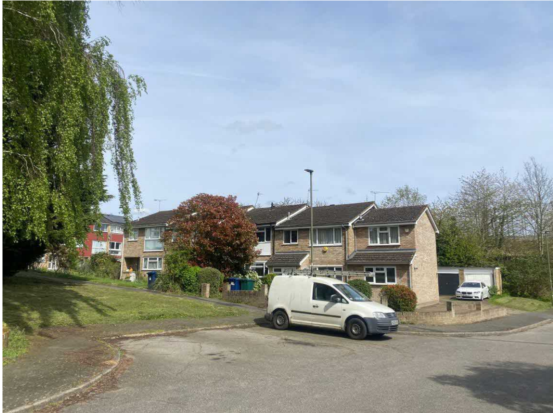
FRONT OF 52 - 58 CROMER ROAD
