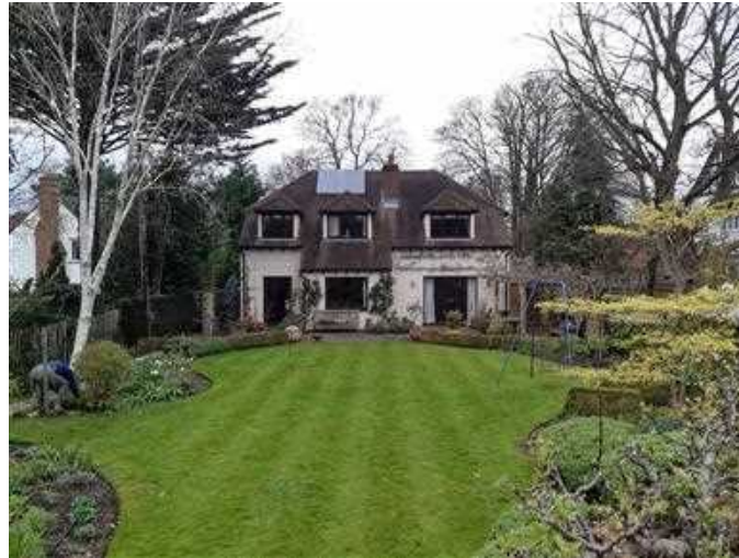
From bottom of garden looking north towards the south facing roof pitch on which up to 10 (approx.) PV panels to be fitted (replacing existing thermal panels).
