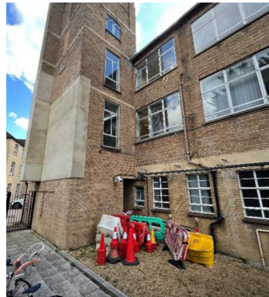
North - Existing condition
