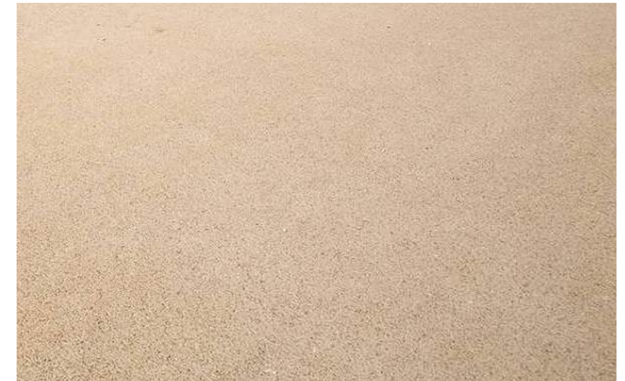
Buff bituminous macadam surface to pedestrian and vehicular areas.
