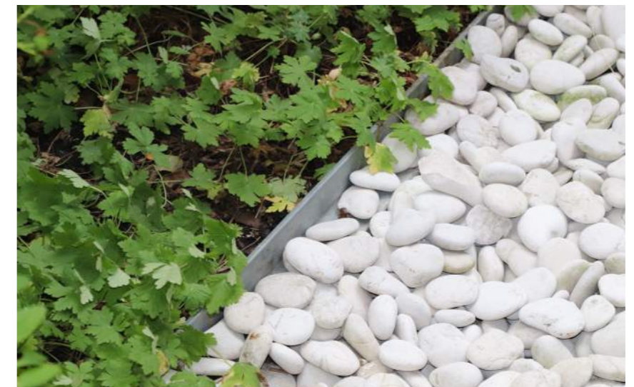
Metal edging and pebble margins to facade interfaces.
