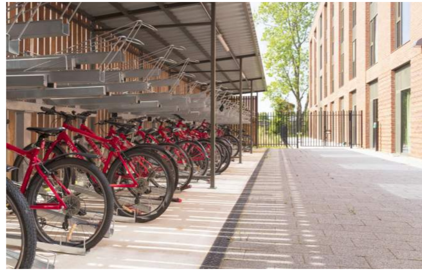
Sheltered cycle storage unit with two-tier storage racks.
