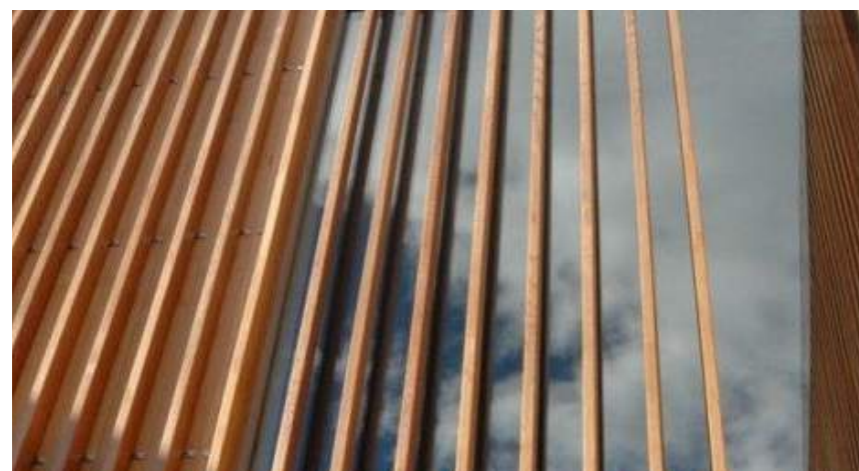
Timber rainscreen and shading example
