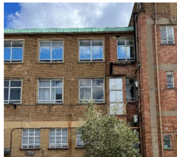
West - Existing condition
