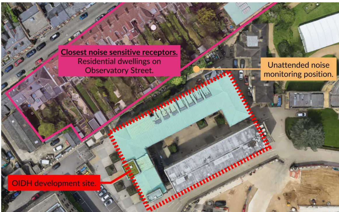
Figure 3: Unattended monitoring position in relation to development site and closest noise sensitive receptors.
