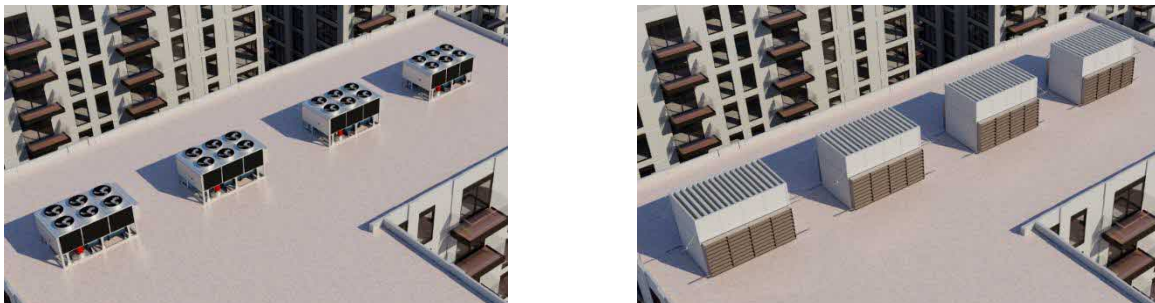
Figure 8: Example mechanical mitigation required on each ASHP. Left – no mitigation. Right – mitigation applied to sides and top.
