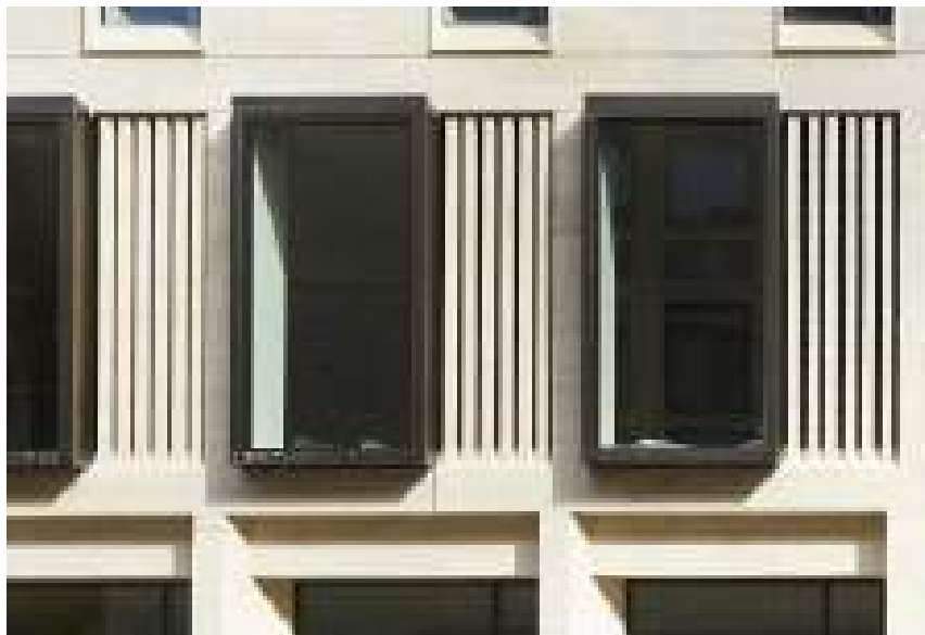
Example of vertical stone baguettes in front of louvres - Cheng Yu Tung Building Oxford
