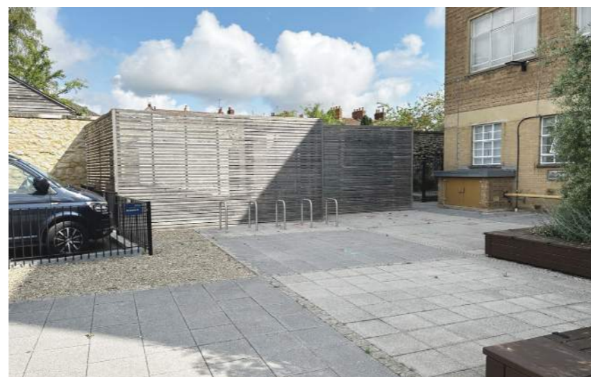
Acoustic fencing enclosure around existing sub station.
