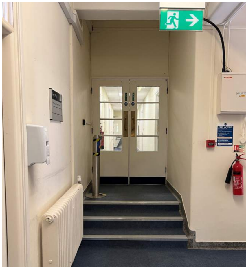
Site Photo Showing Gibson Building SW Corner Level Change (L1)
