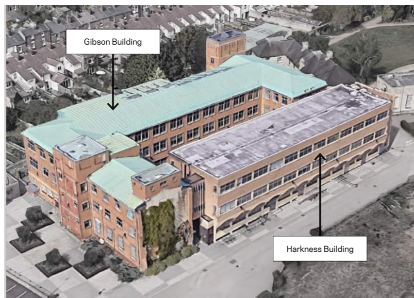
Existing Gibson and Harkness Buildings
