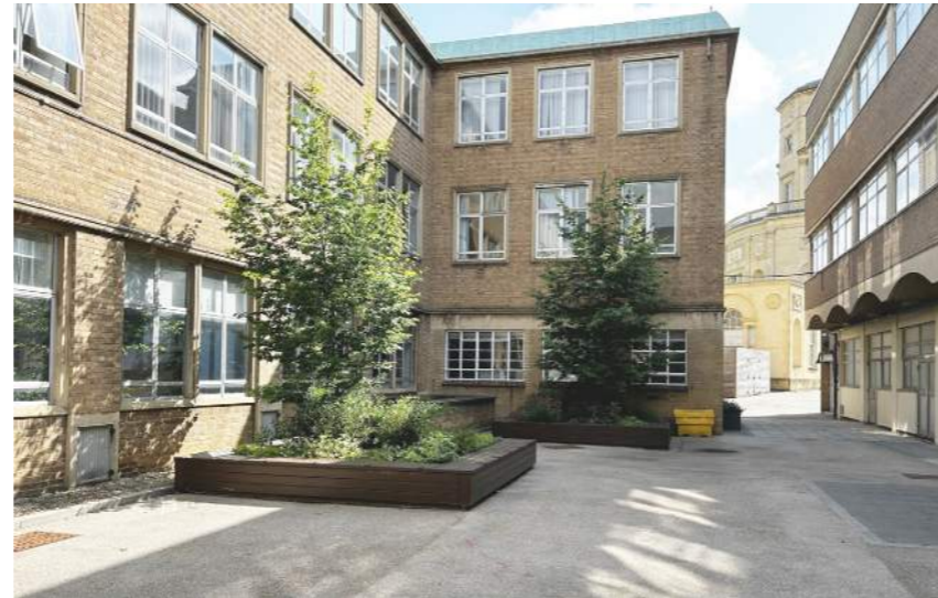
View within central courtyard.
