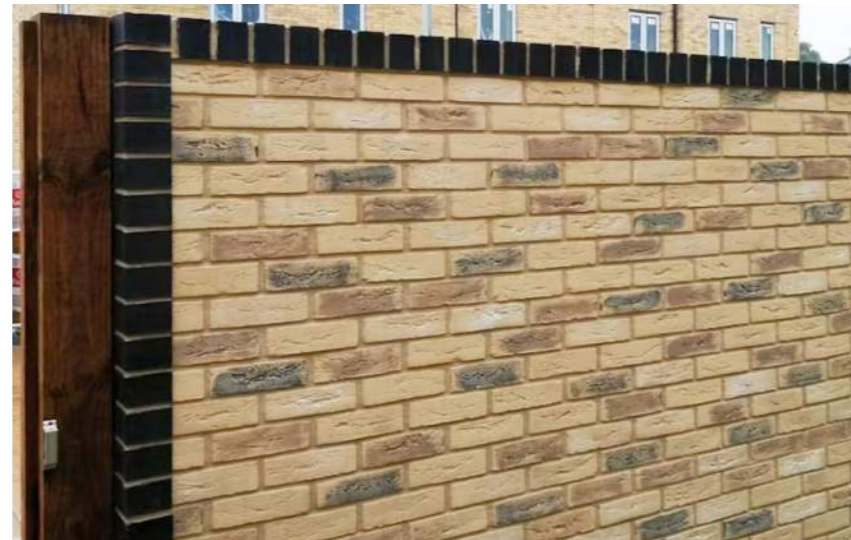
Brick boundary wall to bin storage enclosure.
