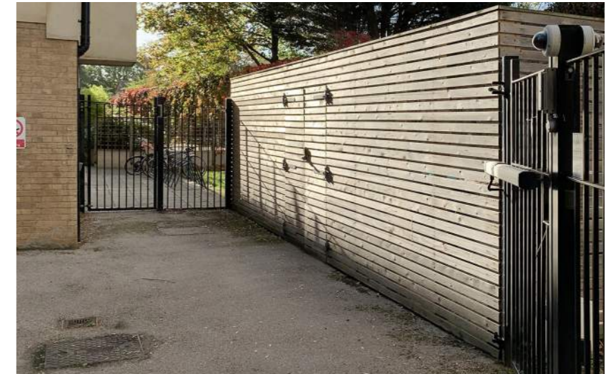
Existing timber fencing and metal gates to rear garden to be retained.
