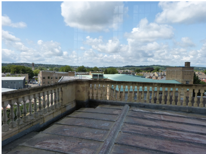
Looking west from inside the lower level of the Observatory tower. The copper roof of the Gibson Building is visible behind and just above the balustraded parapet of the Observatory wing.
