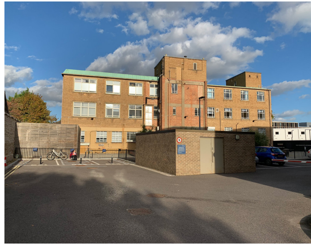
South elevation of the Gibson Building
