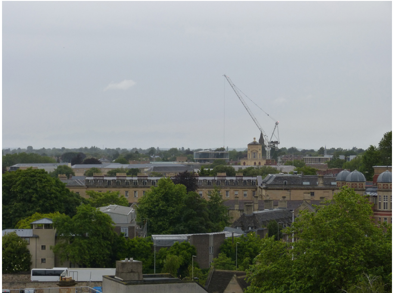
A zoomed in view of the site from St George's Tower (NB: this is not an accurate representation of what the eye sees unaided).
