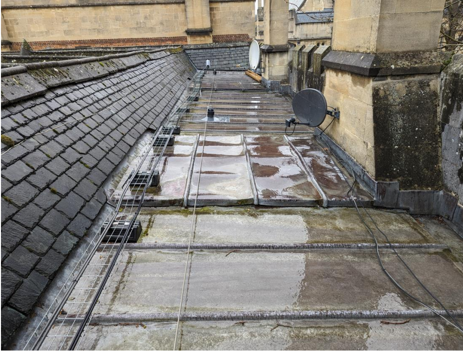
Figure 1: View from roof access door looking West
