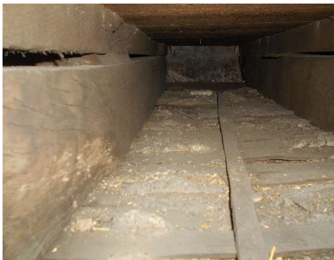
Photograph No 8 – Investigation – Raised Bay d)
