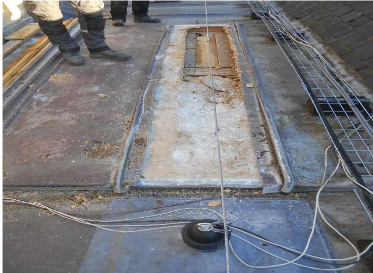
Photograph No 5 – Investigation – Raised Bay a)
