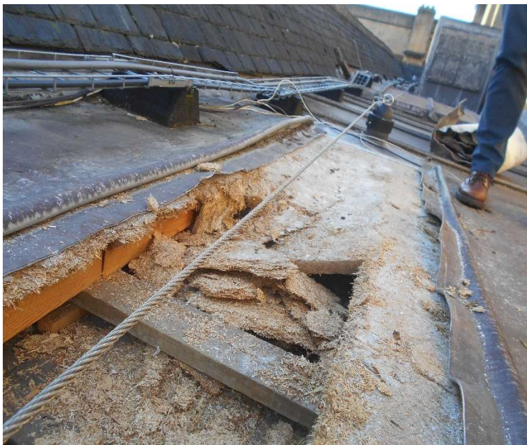
Photograph No 6 – Investigation – Raised Bay b)
