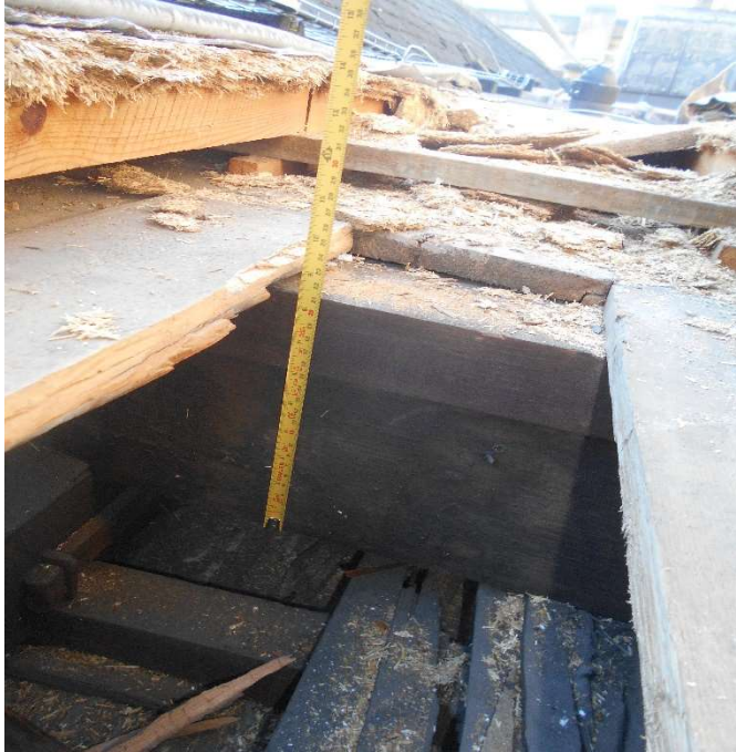
Photograph No 7 – Investigation – Raised Bay c)
