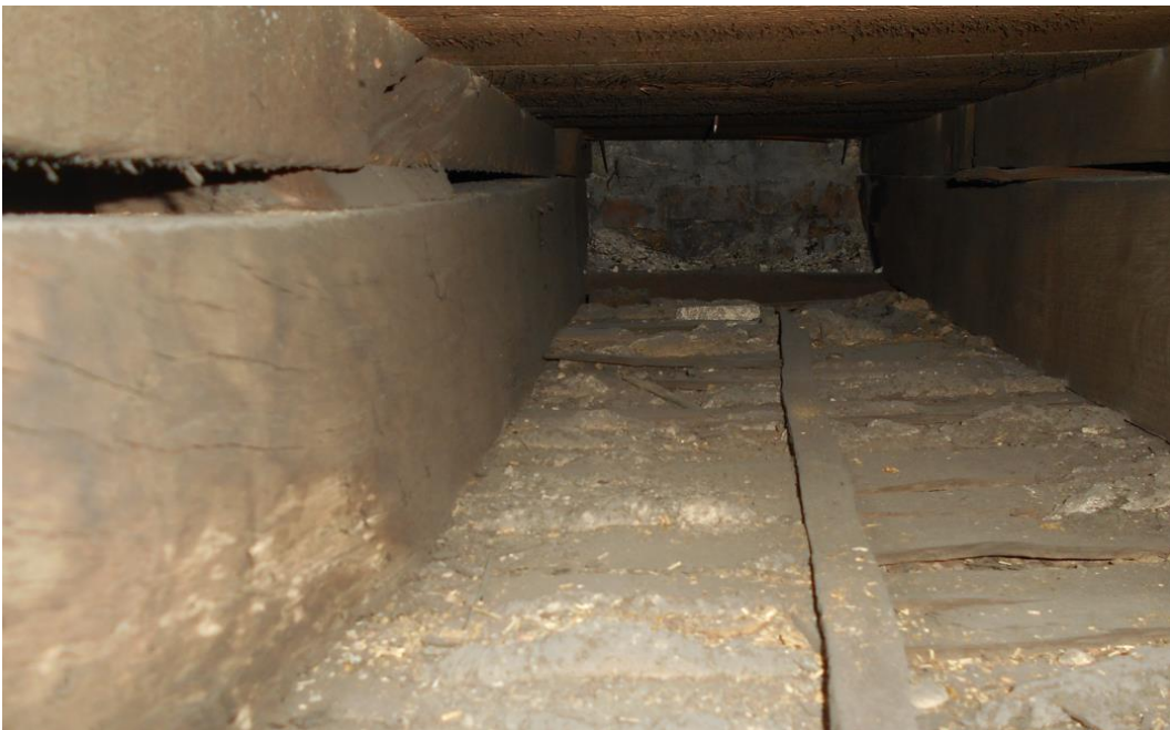
Figure 2: Photo provided by Sidleys showing flat roof structure
