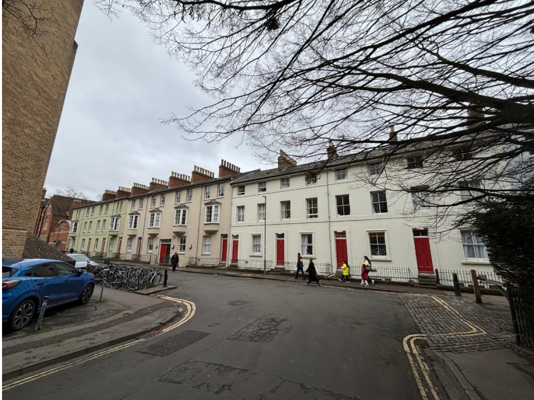
Figure 2 – Front elevation of Lincoln Hall, Museum Road
