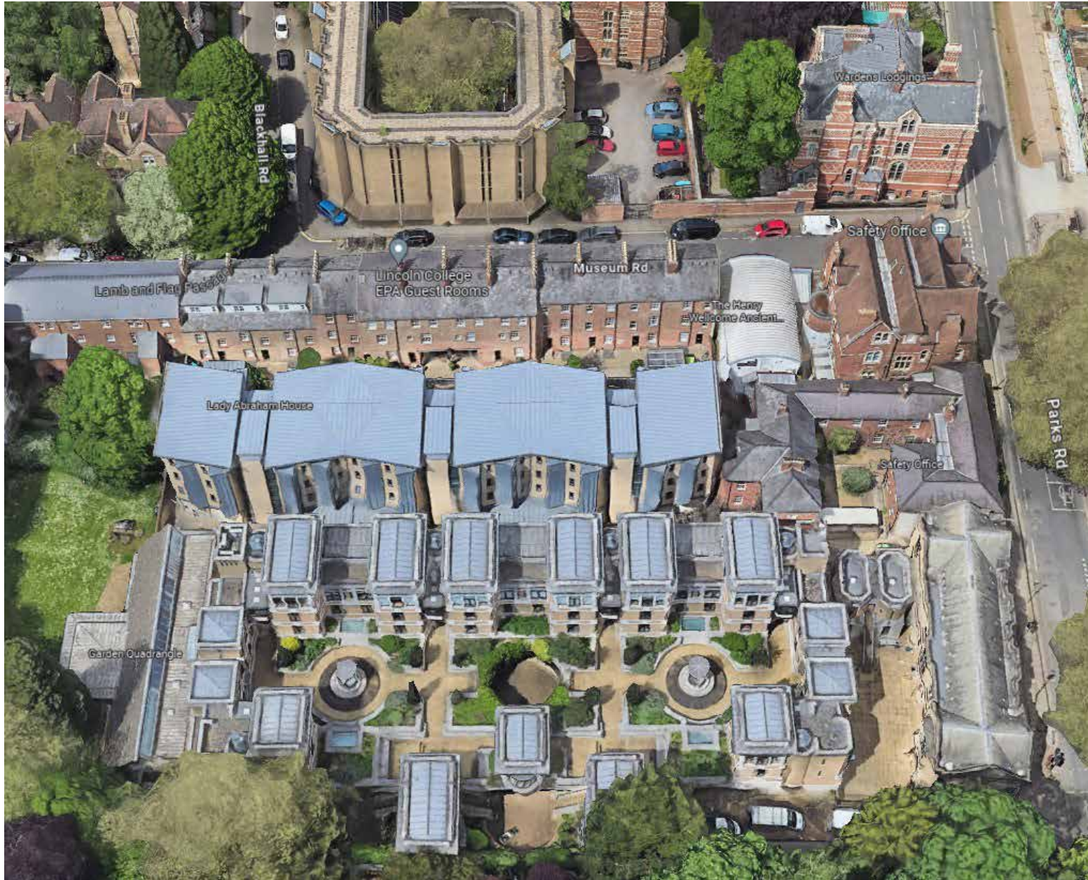
3.5 Aerial view of EPA Science building and Garden Quad in relation to the rear of nos. 1-23 (odd) Museum Road, looking north (Google Maps)
