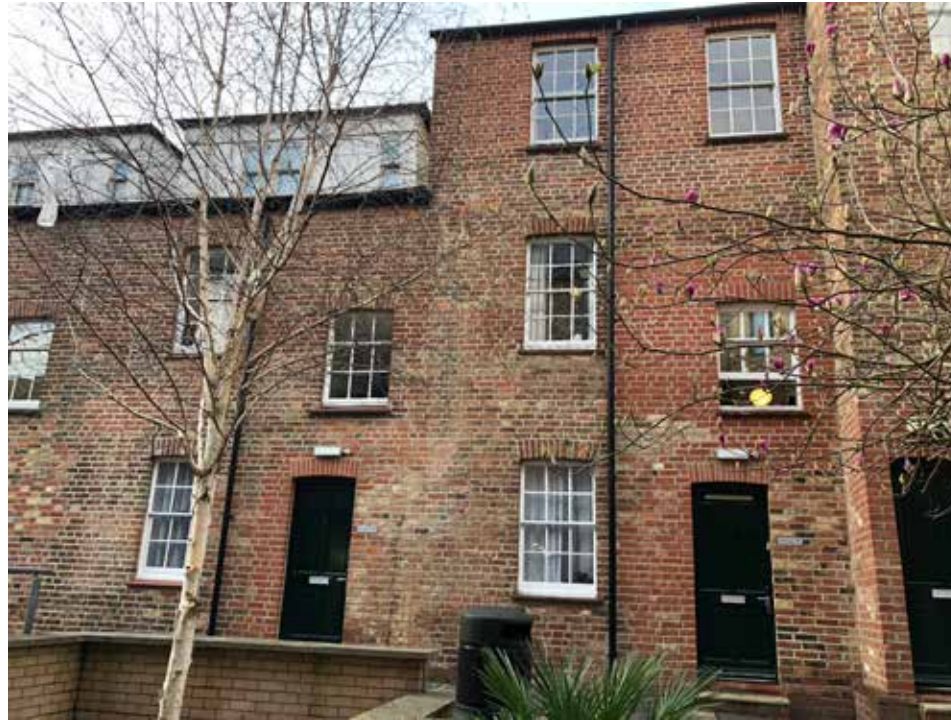
3.13 Rear elevation of nos. 17-19 (DIA)
