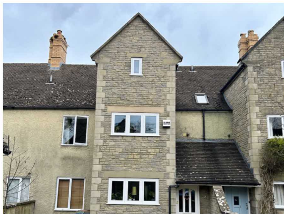
Figure 14. Front elevation / south façade of 4 Lewin Close.
