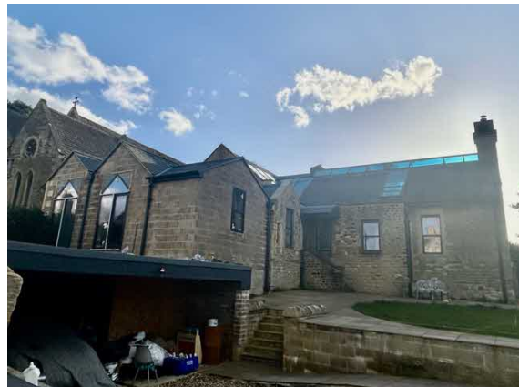
Figure 11. St. James' School (7 Beauchamp Lane) is across Beauchamp Lane to the west of 3-5 Lewin Close. It features a semi-glazed roof with a broken ridge line as well several extensions of various size and height.
