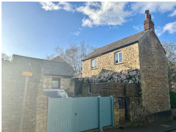
Figure 12. The cottage (5 Beauchamp Lane) is north of the school. It has been extended with two additional structures forming a roof with 4 different ridge heights.
