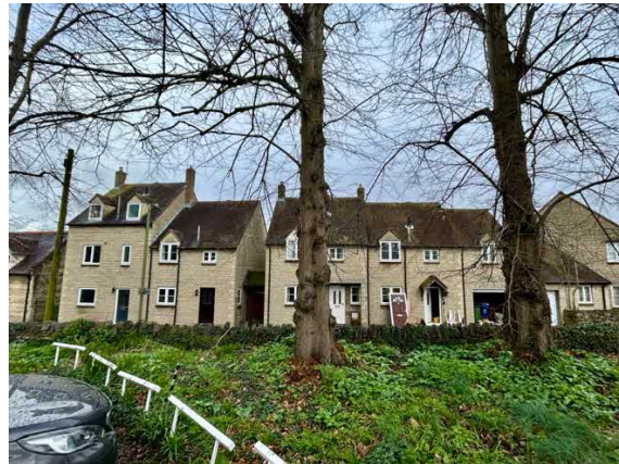
Figure 9. 15-22 Beauchamp Lane as an example for the typical unequal ridge heights in the conservation area.
