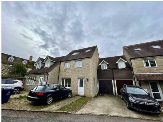
Figure 8. 6-8 Lewin Close as an example for the typical unequal ridge heights in the conservation area.
