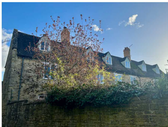
Figure 16. 3-5 Lewin Close has six modern dormers on the north facing roof, which suggests these were installed after the building was listed.
