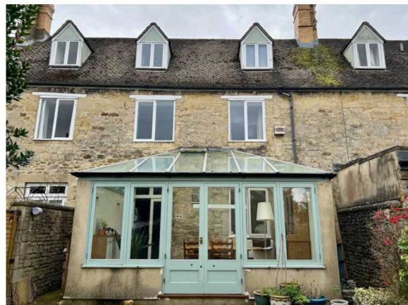
Figure 15. Rear elevation / north façade of 4 Lewin Close.
