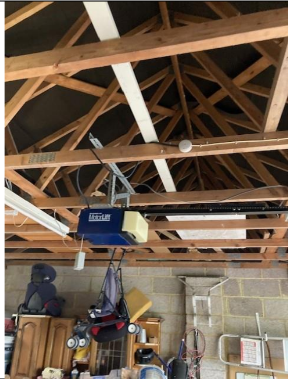
Photo 6: Internal structure of roof
