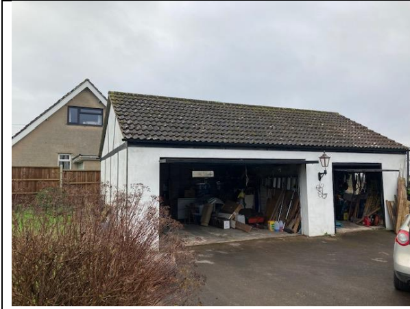
Photo 1 – West face of Garage
