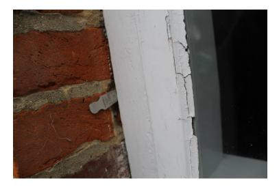
Significant voids between the frame and the masonry. Also, poor condition of the putty
