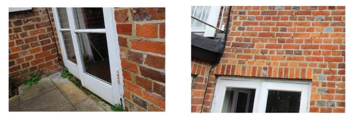
Left - cracked glass, lack of weather bar or any projecting cill. Rusting hinges.
