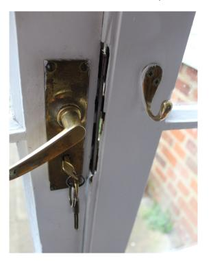
Even closed, there was such warping of these doors that they could not be closed. When timber has warped like this it is not only a sign of a poorly made item, but also it is extremely difficult to rectify.
