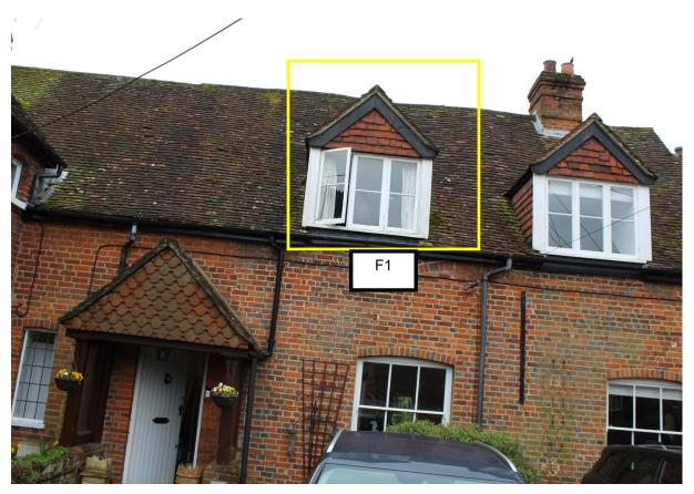
Item F1 is a window - a triple casement window, with two openers and fixed central. The casements are subdivided into two large panes, and the window which is proposed for replacement is of a type with the corresponding one next door.
