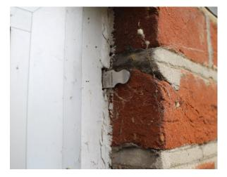
Silicone mastic, smeared over the frame and the masonry - with nothing behind. The taper gauge makes it clear there was a void of at least 150 mm behind the silicone - this shows the poor installation.
