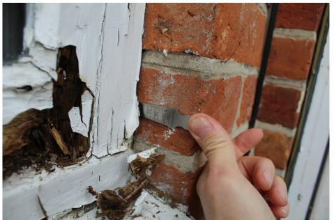
As elsewhere, significant voids between the masonry and the timber frame. This is a major contributor to the poor condition.
