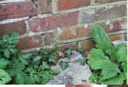
The presence of the plastic "DPC" helps date when this doorway was infilled - likely post 1960. The reasoning for this being that the plastic DPC was uncommon prior to this, and the aluminium window (R1) is thought probably circa 1960.
