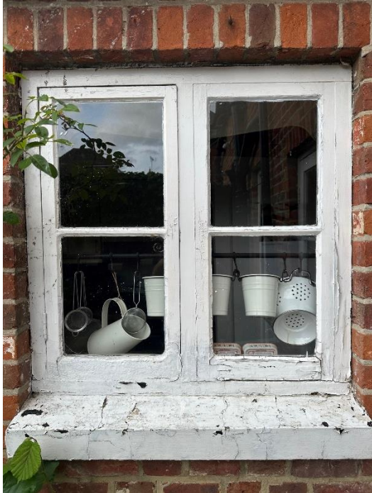
Fig 1.5 Ground Floor Rear Side Elevation window replacement. Existing painted concrete cill to be sanded & redecorated
