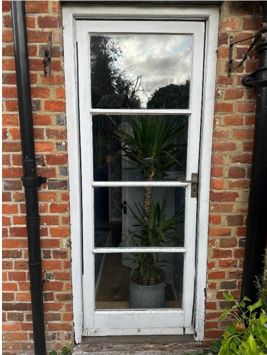
Fig 1.4 Ground Floor Rear Elevation Patio single door set & hardwood threshold replacement
