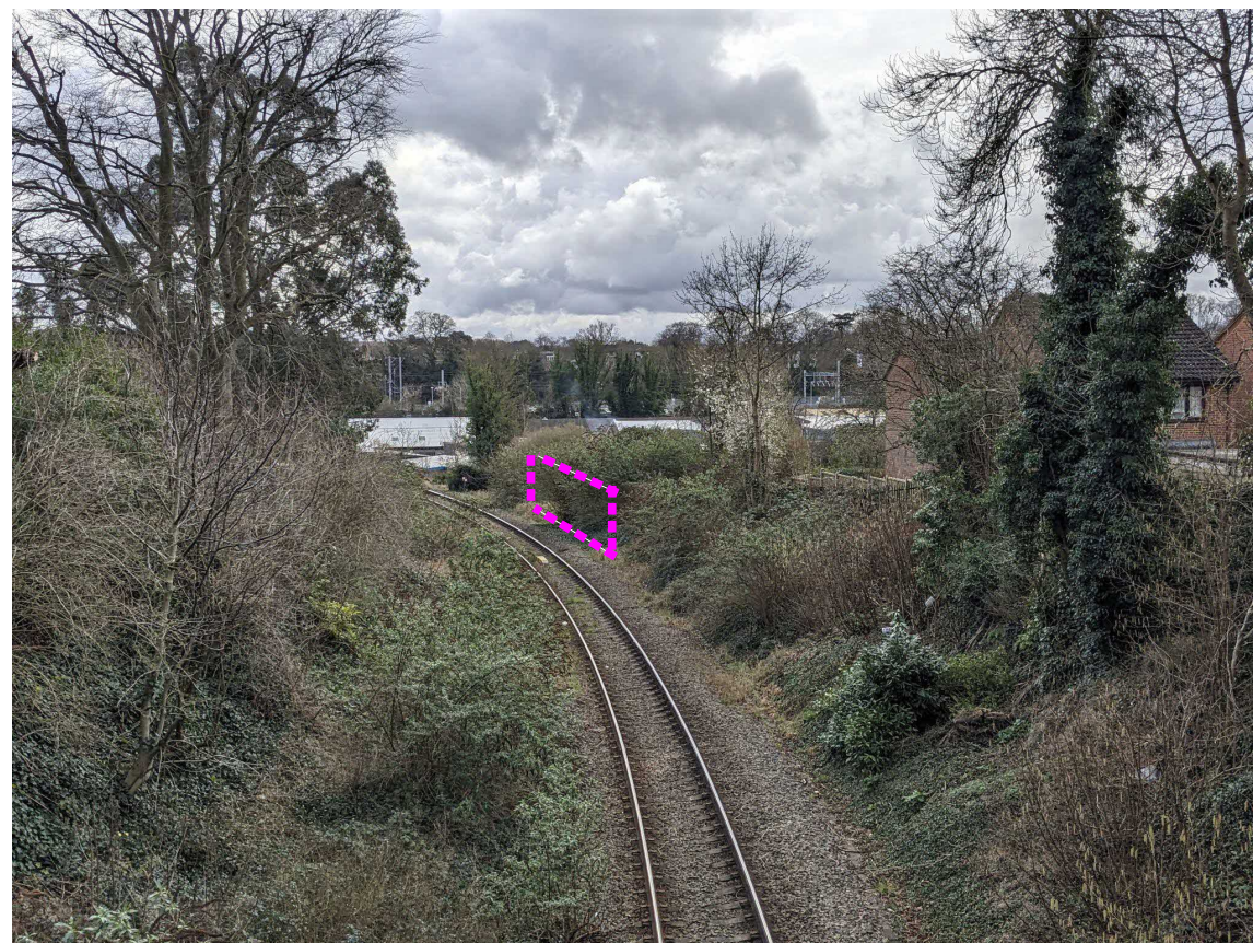
View from Grenfel Rd road bridge
