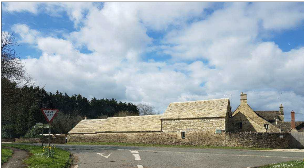
Fig 3 Conversion at bottom of lane
