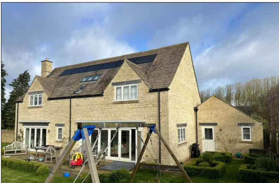
Fig 2 Rear of house
