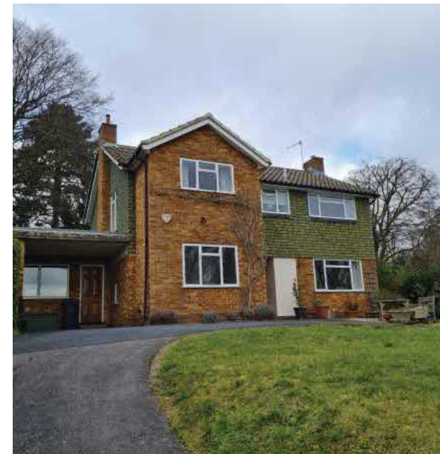
Existing south elevation with yellow brick and green tiles
