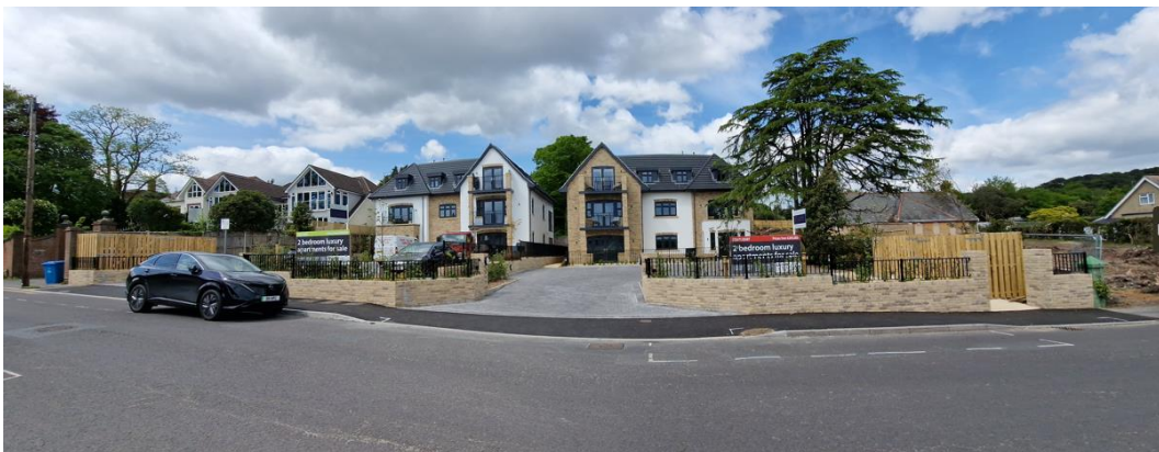
Existing flatted development at nos. 13 and 15 Danecourt Road
