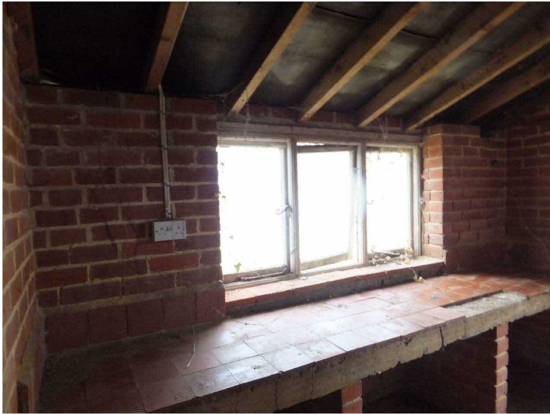
Fig 9 Internal view of rear of West lean-to
