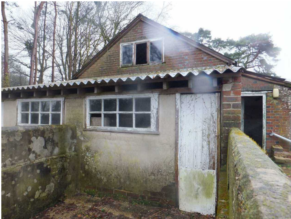
Fig 16 Rear elevation of Rear lean-to
