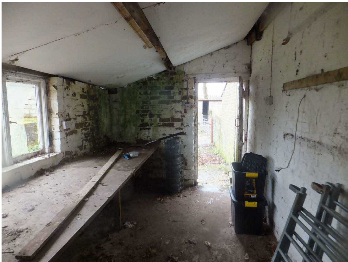
Fig 14 Internal view of rear wall of East lean-to
