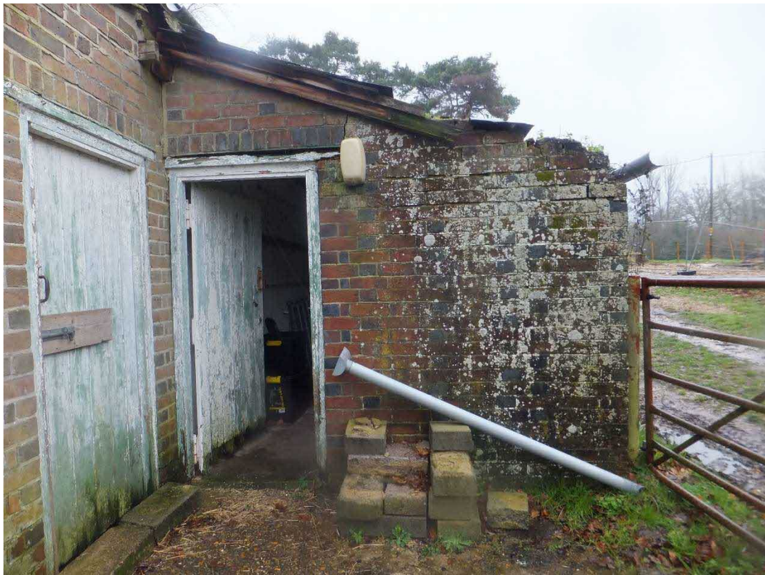
Fig 12 Rear elevation of East lean-to
