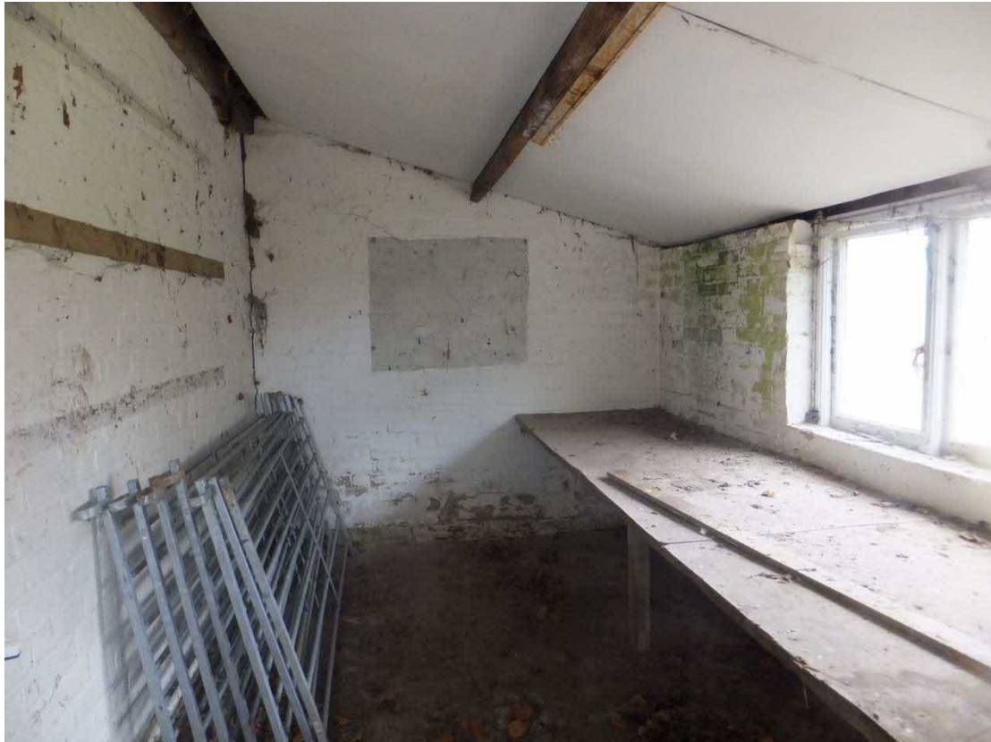
Fig 13 Internal view of front wall of East lean-to
