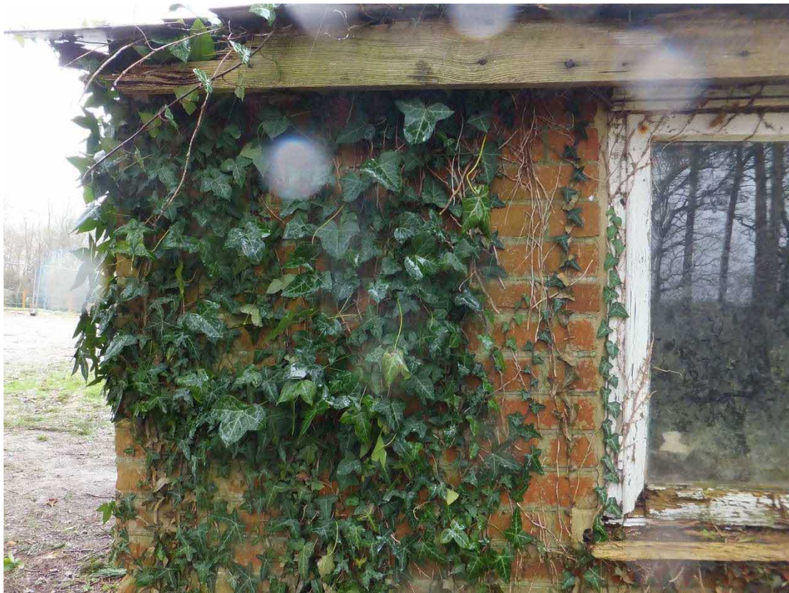
Fig 22 West lean-to –external view
