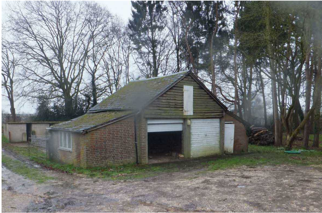
Fig 1 North/Front Elevation of Pig Barn
