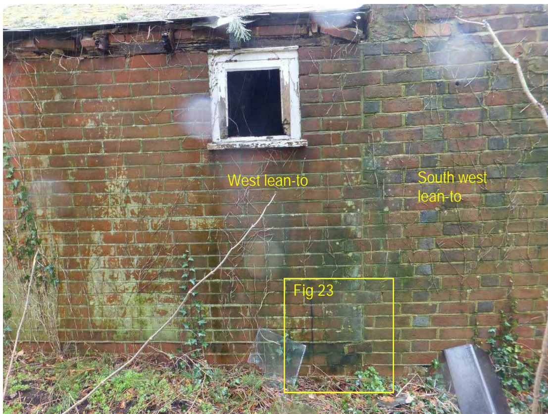
Fig 23 West lean-to –external view
