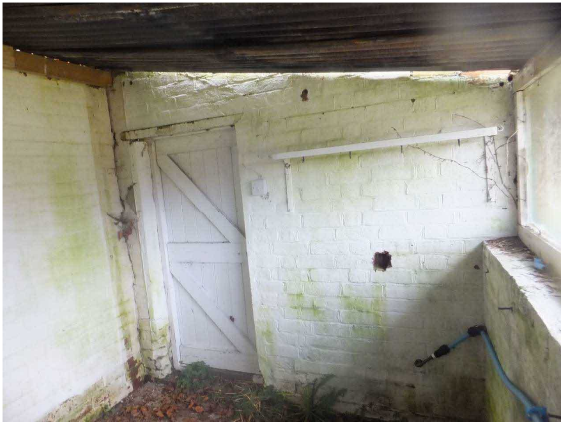
Fig 20 Internal view of Southwest lean-to –showing doorway to Rear lean-to
