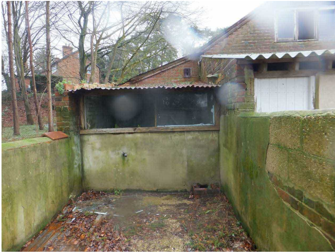
Fig 19 Rear elevation of Southwest lean-to
