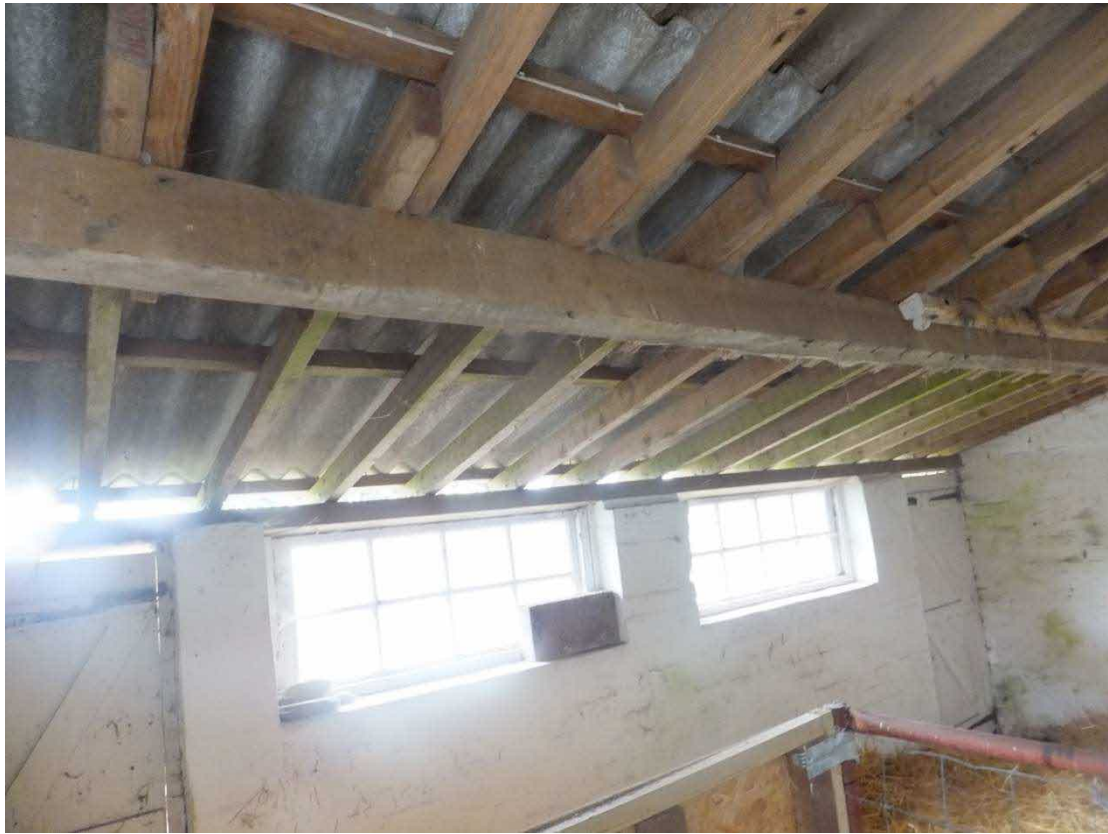
Fig 17 Internal view of Rear lean-to
