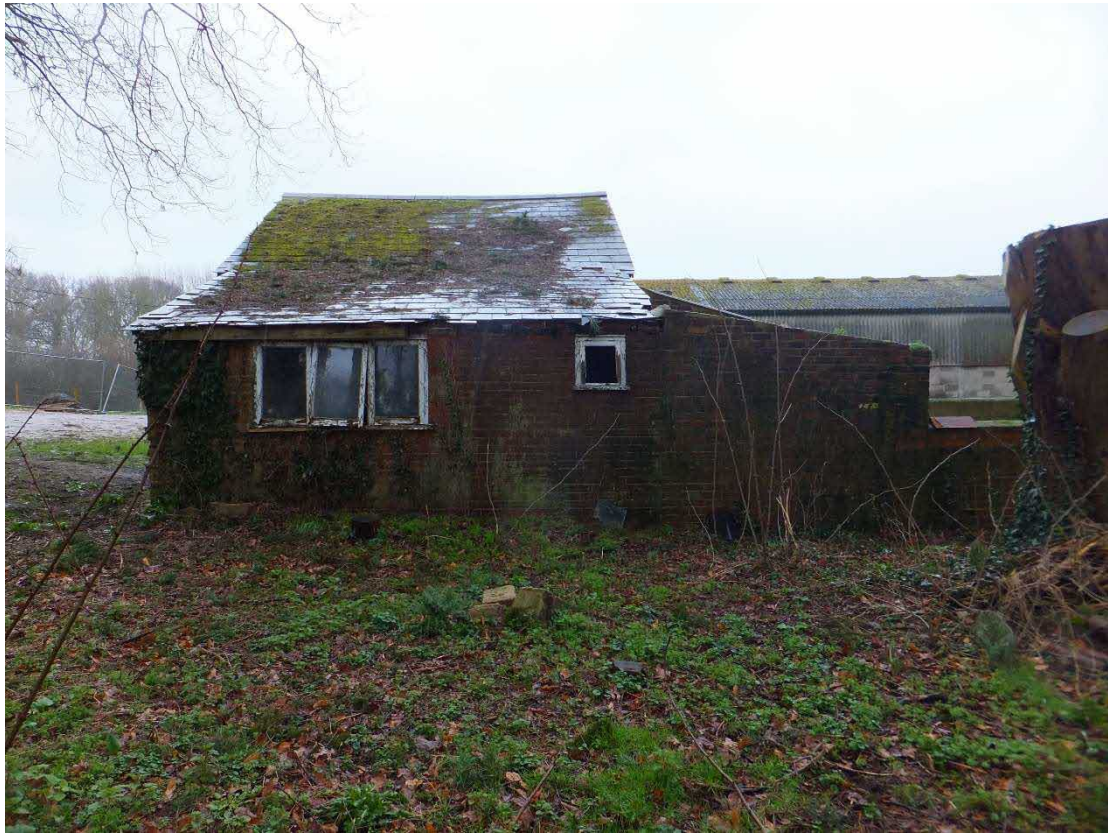
Fig 7 West elevation showing lean-to
