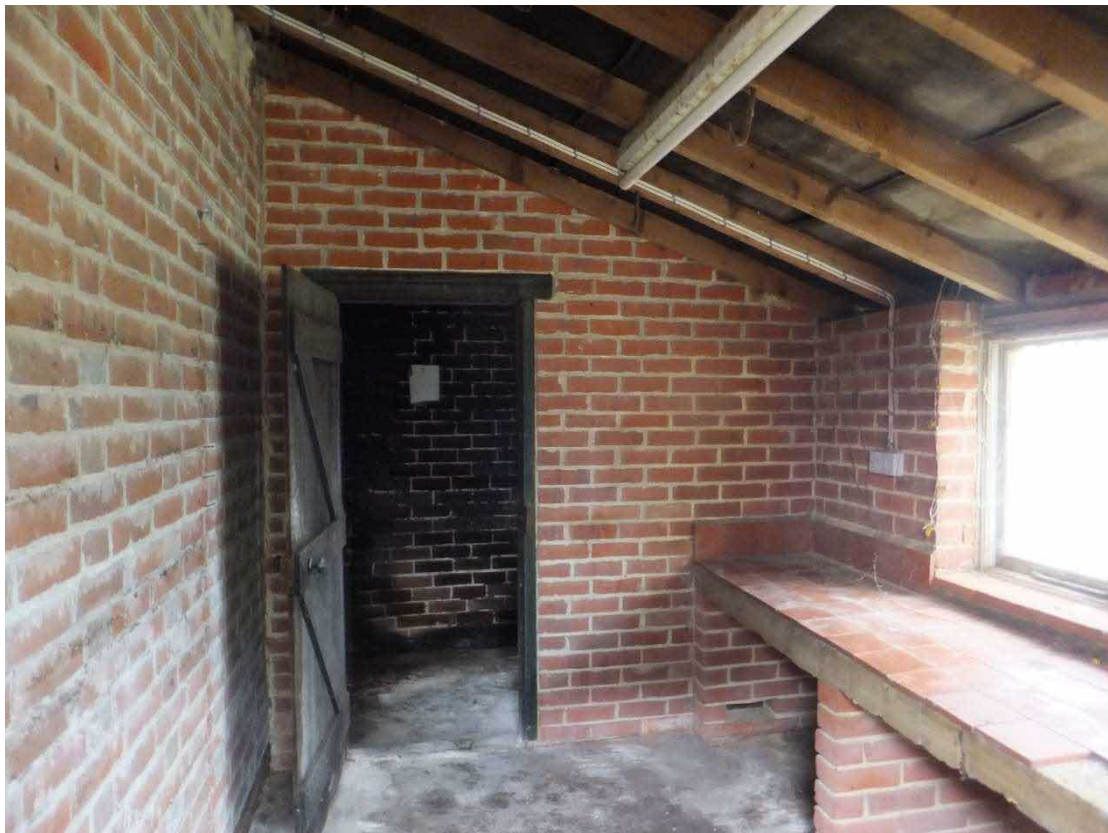
Fig 8 Internal view of rear of West lean-to
