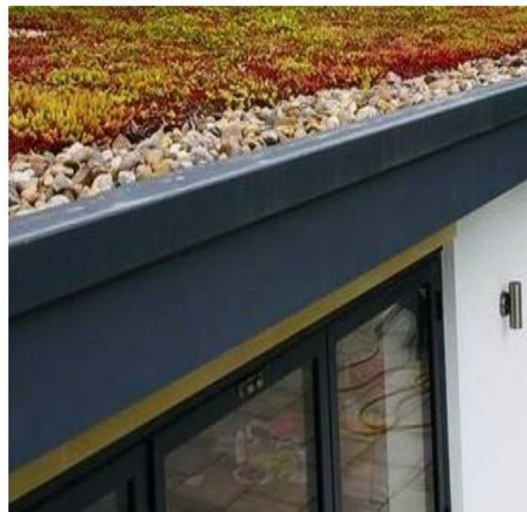
Sedum roof behind metal fascia
