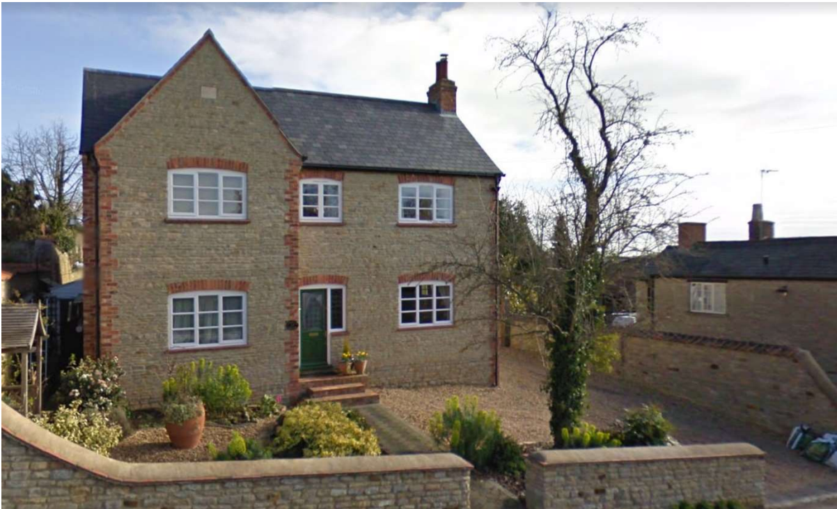
5 - 20 Church Green - Looking North
