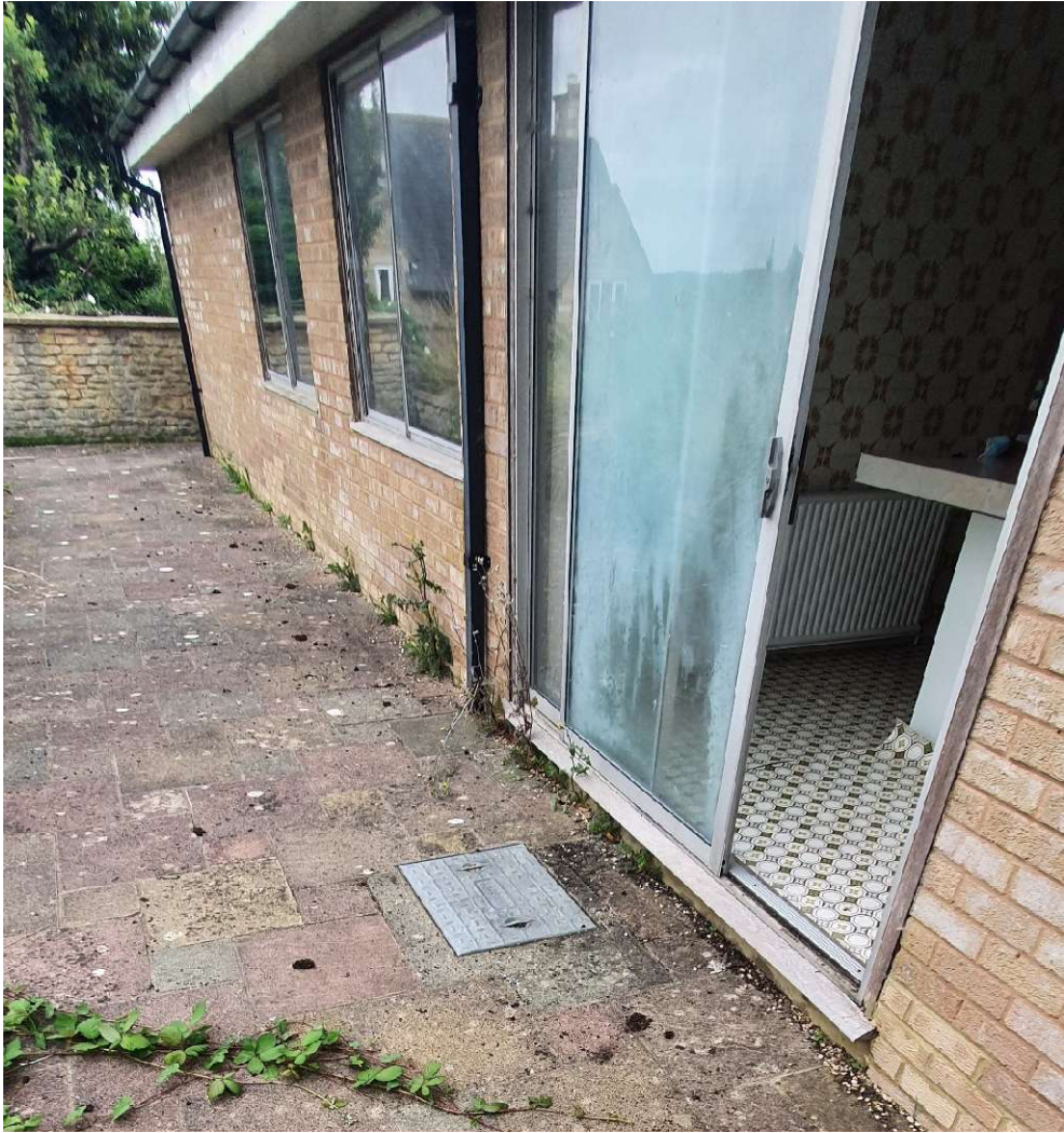
3 - Existing Manhole under proposed extension to be relocated
