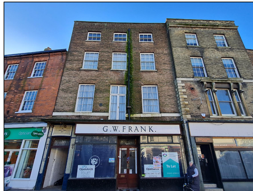
FULL FRONT ELEVATION OF PROPERTY
