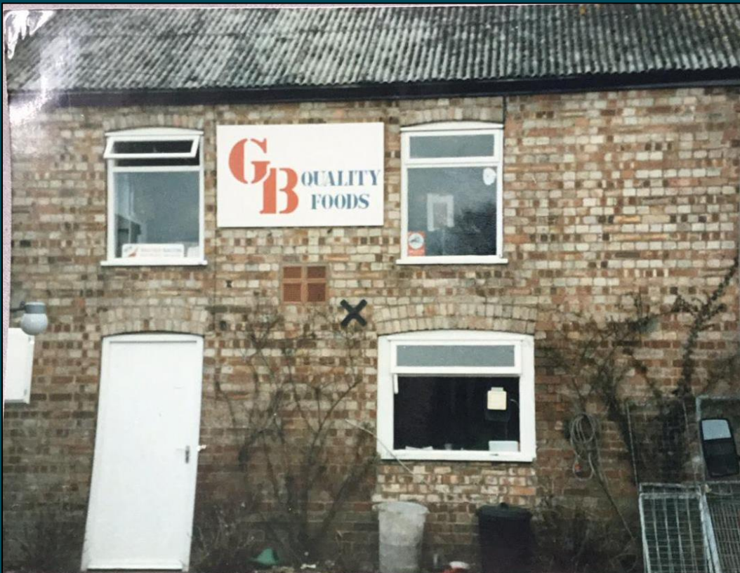
Fig.3 – Photo Showing pre-existing window to be reinstated.
