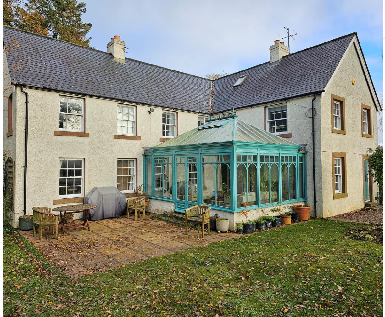
Fig 02-A Existing Rear of Property
