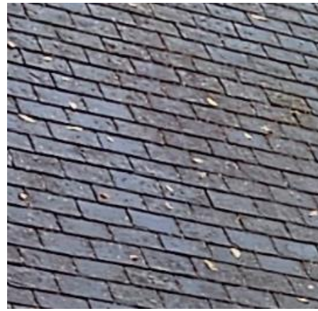
Fig 05-C Slate Roof to Front Extension
