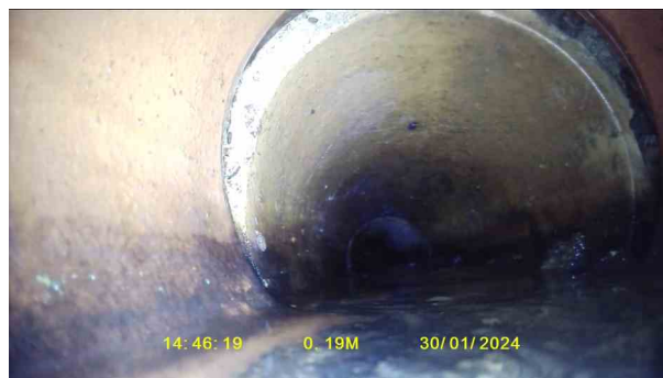
OutfallX_6e46a544-d1a2-496c-aa92-881a1830dace_20240207_144035_842.jpg, 00:00:22, 0.19 m Open joint, medium
