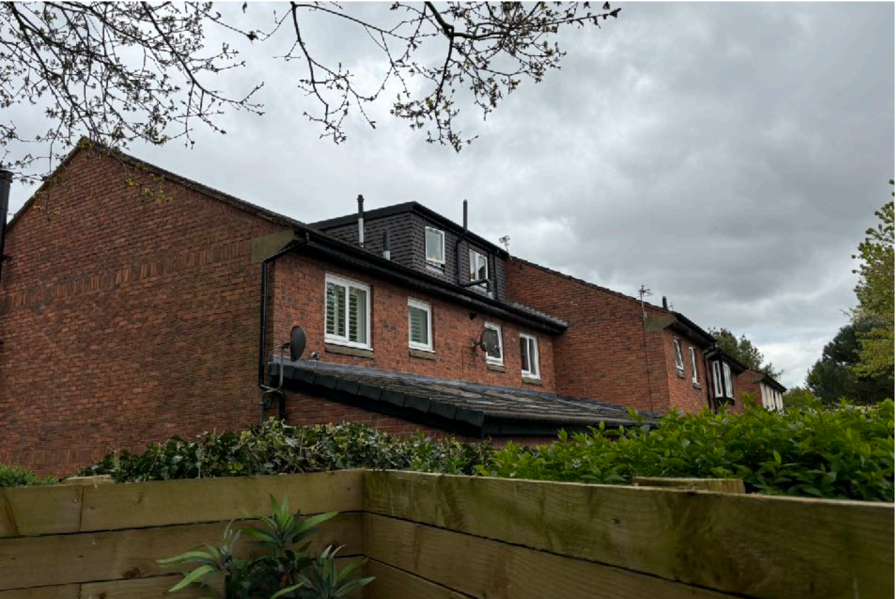
Plate 3: Modern houses to rear, with dormer.
