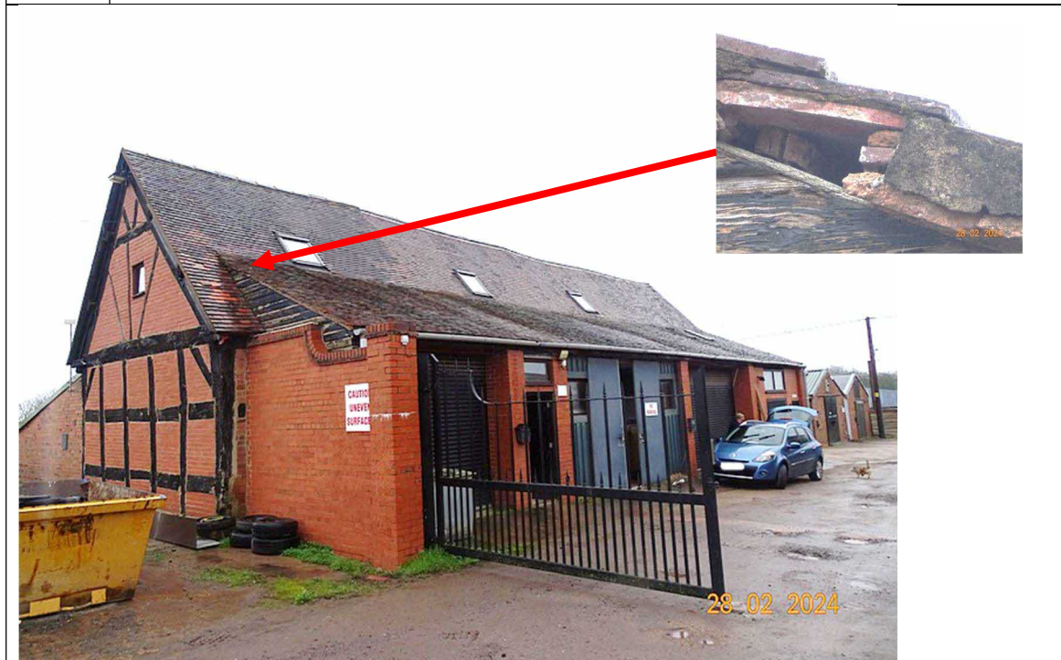
Fig 4. Describing southerly face (front) of building and the side extension enclosing entrances and roller shutter doors. Inset photo describes missing mortar on verge giving potential access for roosting bats.
