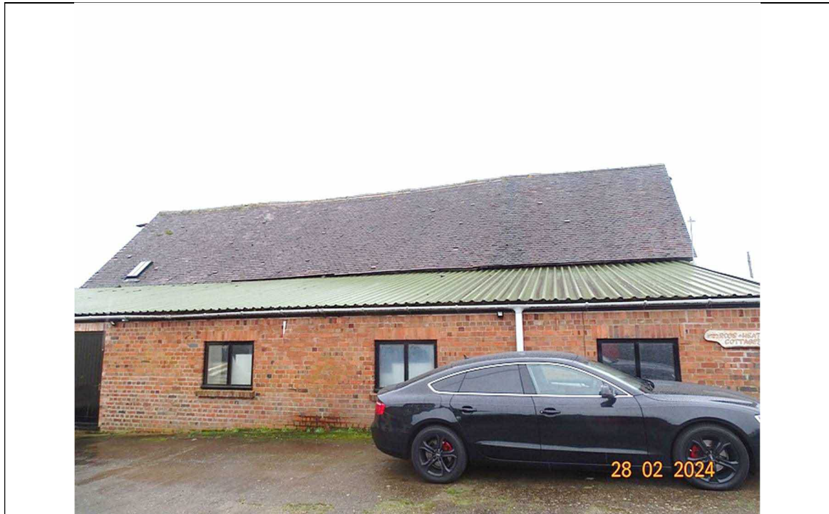
Fig 1. Describing north face of building and rear extension.
