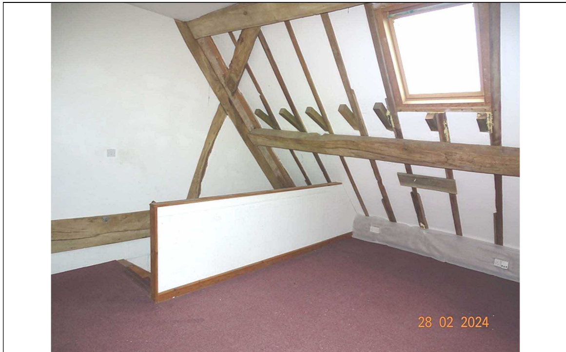
Fig 11. Describing 1 st floor of westerly compartment, note rafters for front extension.
