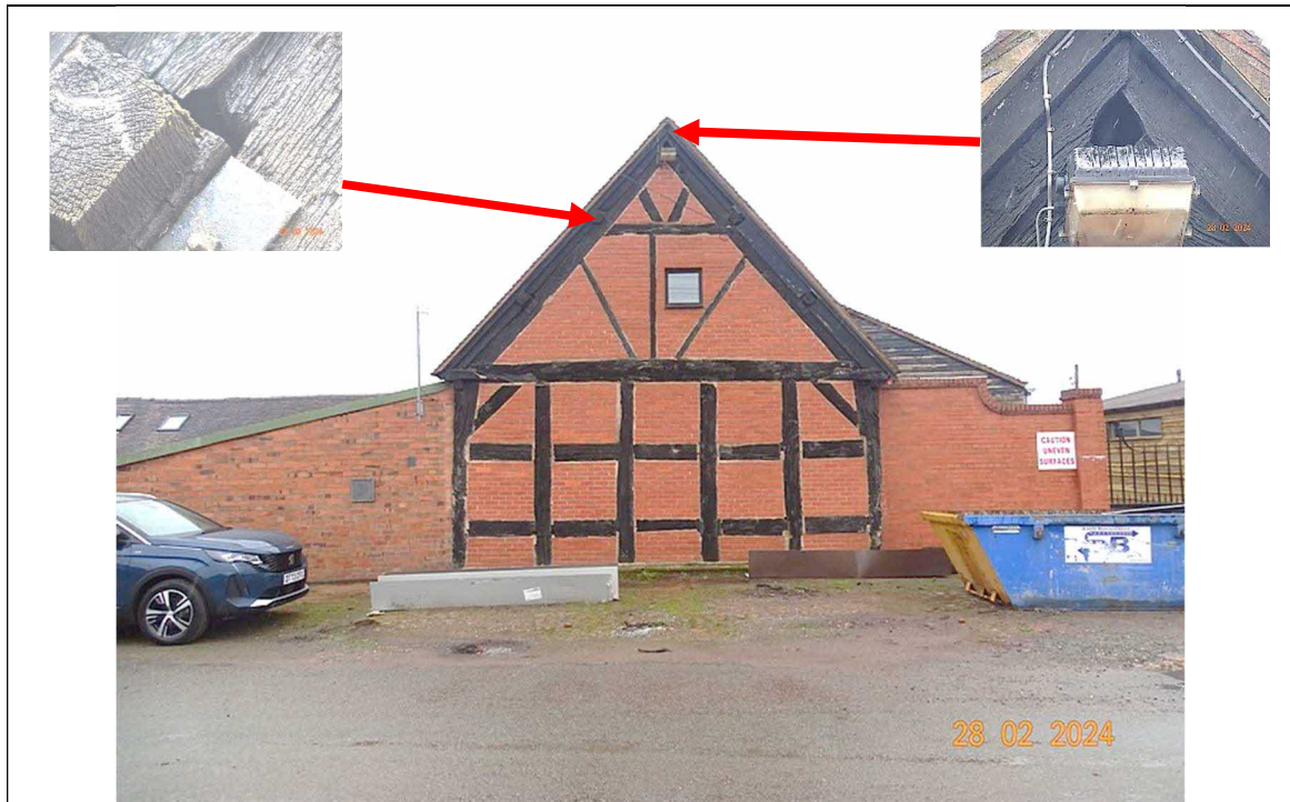
Fig 3. Describing west gable. Inset photos describe potential roosting places for bats.
