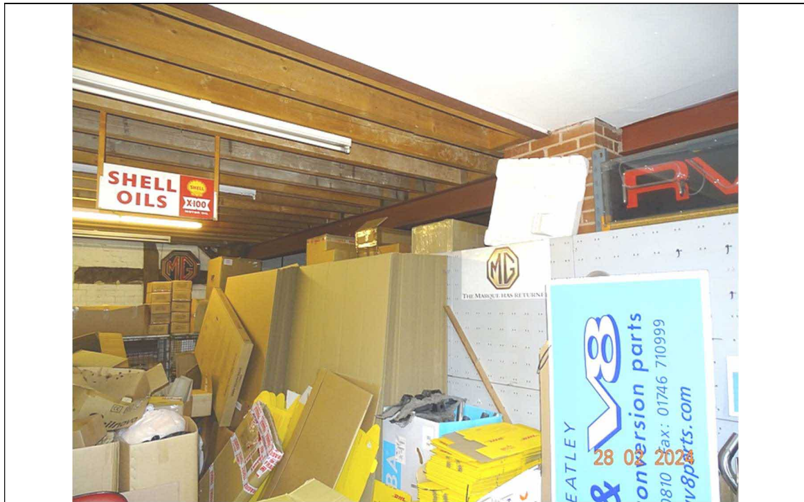
Fig 13. Typical view of central compartment on ground floor.
