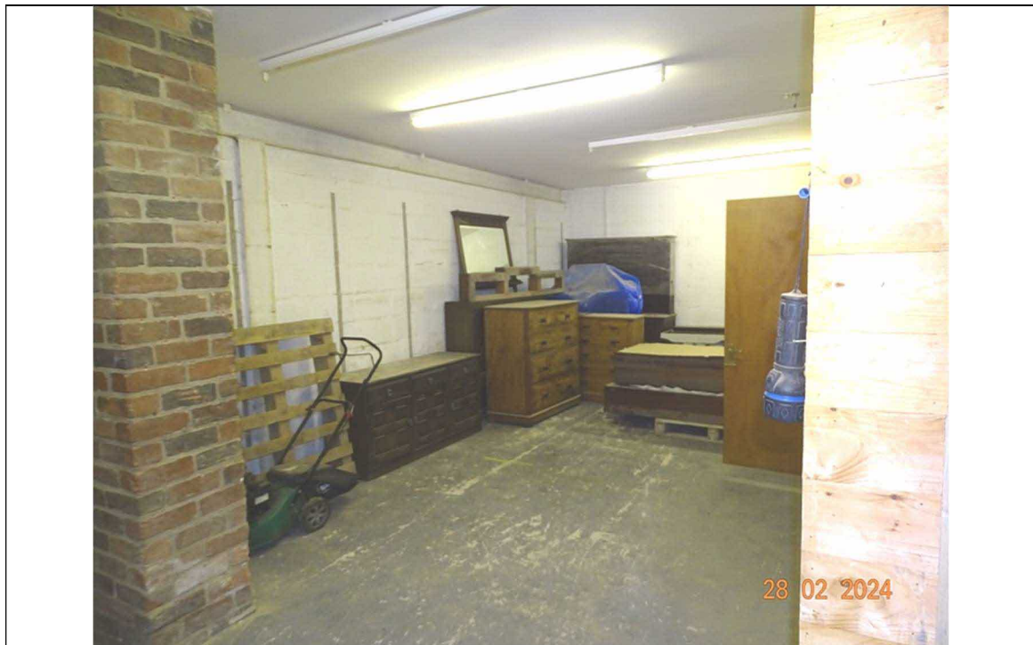
Fig 9. Describing ground floor of westerly compartment.
